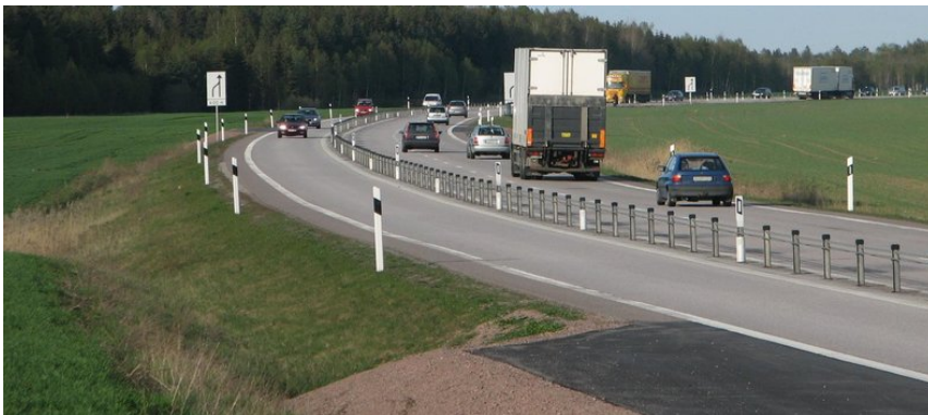
(c) Wire road safety barrier
