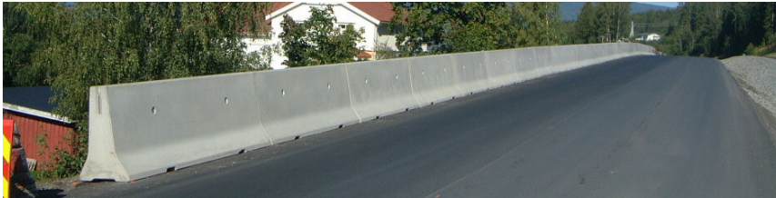
(a) Concrete road safety barrier
