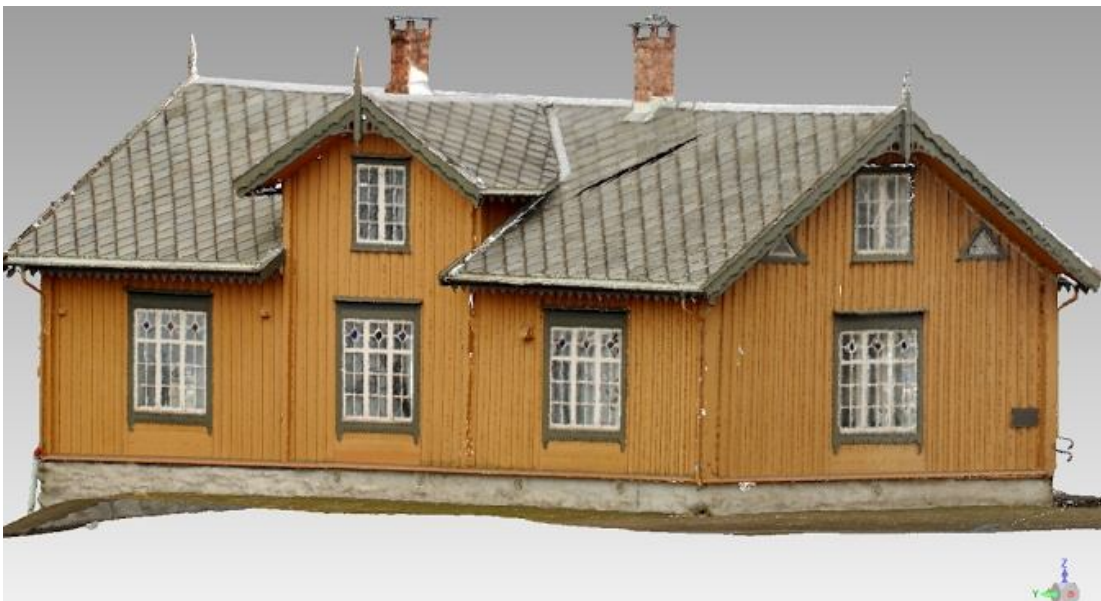
Figure4.3. Østre Gløshaugen building from the north-west side.
