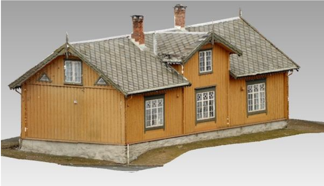
Figure 4.2. Østre Gløshaugen building from the north-east side.
