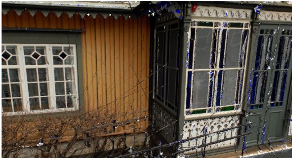
Figure 3.84. Error after importing and texturing 3D model of the house in RiSCAN PRO.
