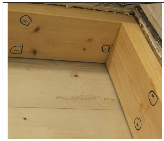
Figur 16: To parallelle skruer i vegginnfesting, vegg 2 2014.
