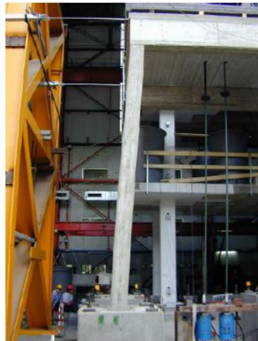
Figure 4.9: Cover spalling and maximum deflection from the 0.80g test (Ferrara & Negro, 2003).
