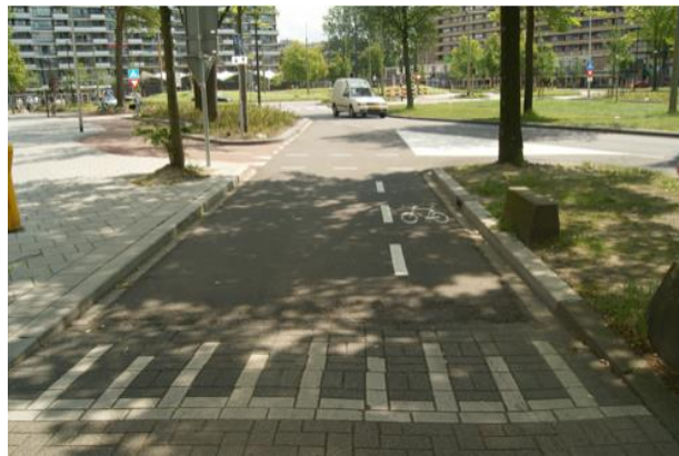
Figure 3: Marked Contraflow on driveway off of Martinus Nijhofflaan in Delft (Brown & Demusz, 2013)
