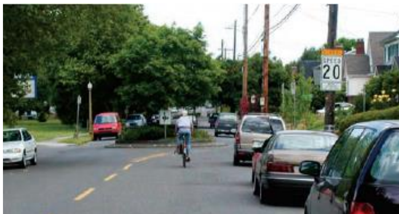
Figure 25: Mini circle slows traffic: creating conditions for Shared Roadway (Oregon Department of Transportation, 2011)
