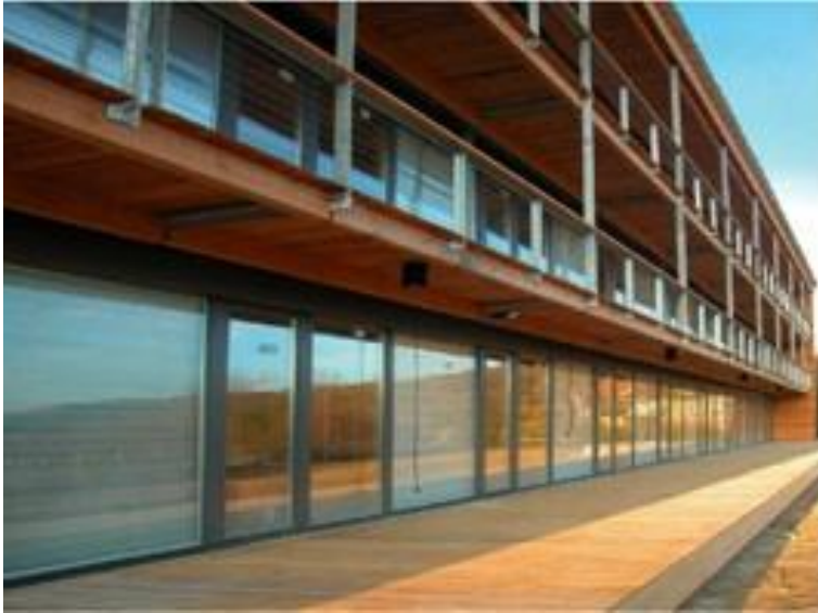
Figure 12 Zero energy office building from Kempen, Switzerland (Cosella-Dörken [22]).
