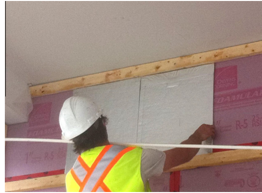
Fig. 12. Installation of VIPs with adhesives [41].
