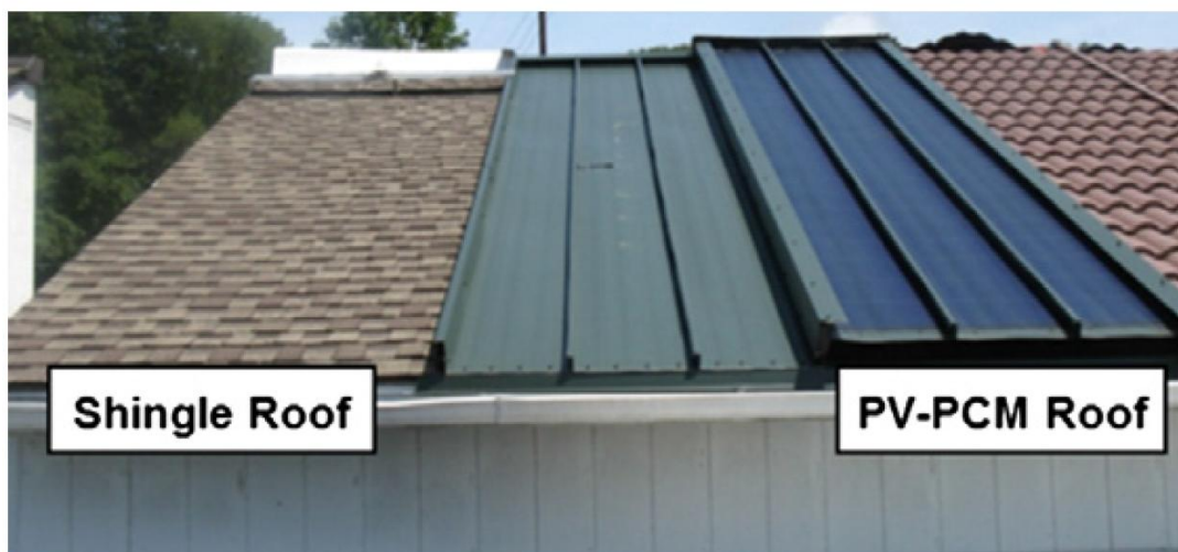
Figure 10 PV-PCM roof (Kosny et al. [60]).
