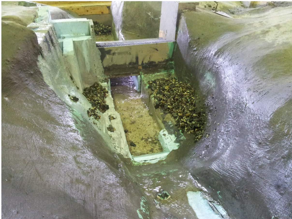
Figur 2.4: Spyling under inntaket.
