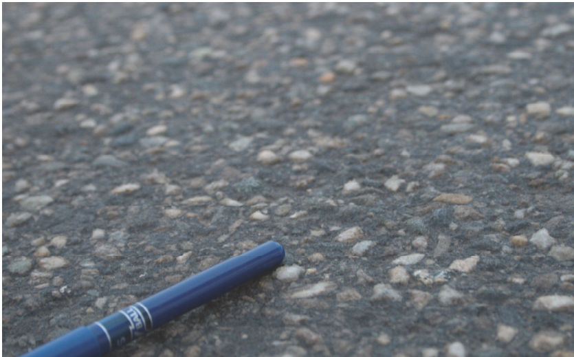
Figure 5.4 The road surface at the observation point.
