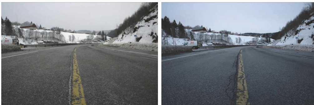
FIGURE 9 The observation point at 09:21 and 16:15.
