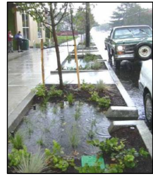
Figur 5-13: Regnbed erstatter sandfang. Hentet fra: (Thorolfsson, 2011)
