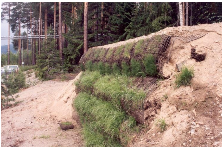
Figur 13: Armert bratt skråning i Hallingtorv (foto: SINTEF).
