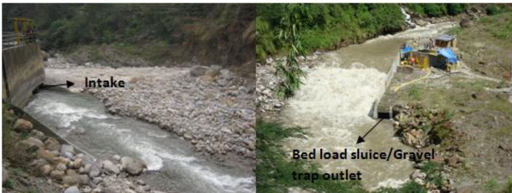
Figure 71 Headworks site of Khudi HPP (Shrestha et al., 2008)
