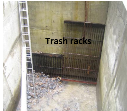
Figure 10 Intake cloggage at Khudi HPP(Shrestha et al., 2008)
