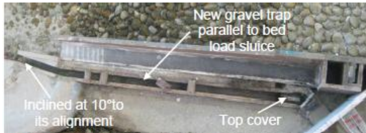
Figure 74 Modifications along the gravel trap on the PHM of Khudi HPP (Shrestha et al., 2008)
