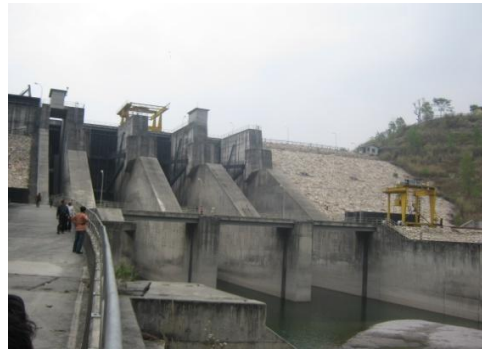
Figure 9 Spillway at Middle Marsyangdi HPP
