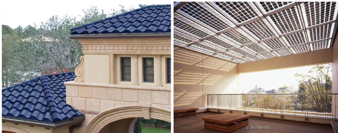
Figure 16. On the left: example of BIPV tiles (Solar Power Restoration Systems Inc, not dated) – On the right : ceiling glas allowing daylight fitted with PV modules (Global Energy Network Institute 2009).
