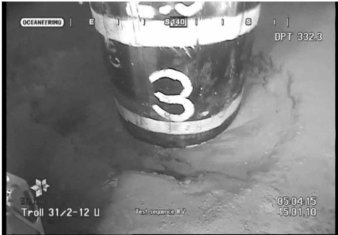
Figure 1-3: Troll well 31/2-12 U Drilling with BOP
