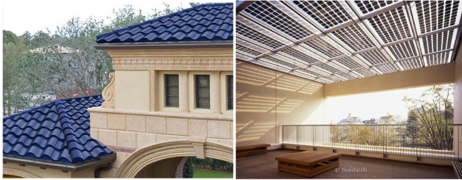
Figure 7: Illustrations of available BIPV systems, from left to right; curved clay-looking tiles and transparent halo ceiling. Source, respectively: Solar Thermal Magazine (2010) [30] and Global Energy Network Institute (2009) [31]
