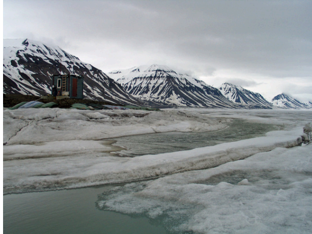
Figure B.87: State of the ice at the tip of the breakwater. The tide crack in the foreground was getting wider. Sea height = -0.7 m – 8 June 2007 (week 23)
