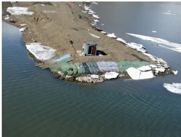
Figure B.110: Aerial view of the breakwater. Photo: Lene Kristensen. Sea height = -0.4 m – 18 June 2007 (week 25)
