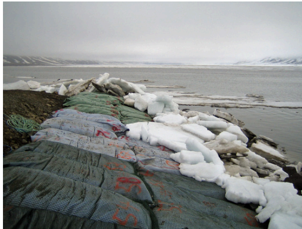
Figure B.117: Ice pile-up at the tip of the breakwater, sea height = -1.0 m – 19 June 2007 (week 25)
