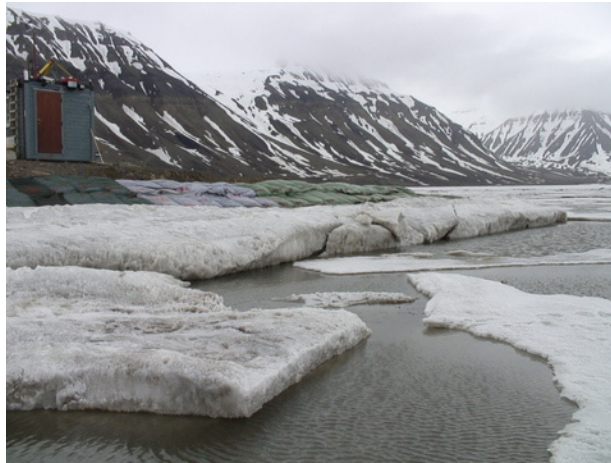
Figure B.92: State of the ice at the tip of the breakwater, sea height = -0.8 m – 13 June 2007 (week 24)
