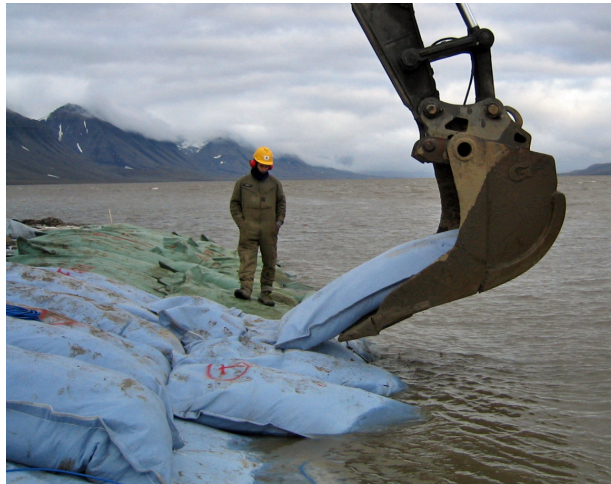
Figure C.12: Installation of a bag
