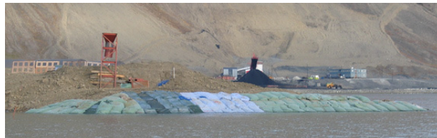
Figure C.8: View of the breakwater after installation of the geosynthetic bags
