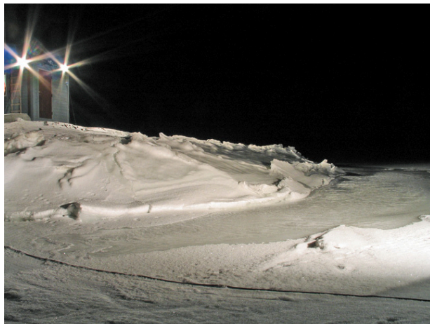
Figure B.45: Pond of surface water along the tip of the breakwater, sea height = -0.7 m – 5 January 2007 (week 1)
