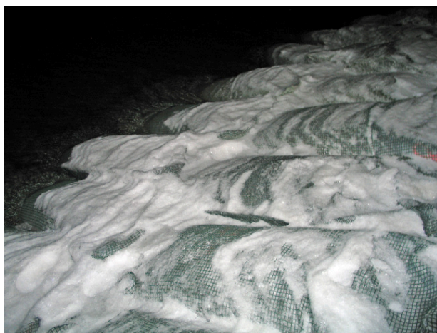
Figure B.27: Ice rubble on the bags, sea height = -0.6 m – 22 November 2006 (week 47)
