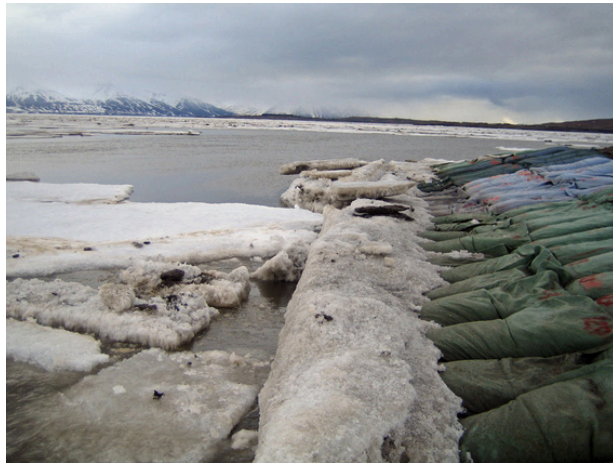
Figure B.107: Drift ice scouring against the lower bags at low tide, sea height = -0.6 m – 16 June 2007 (week 24)
