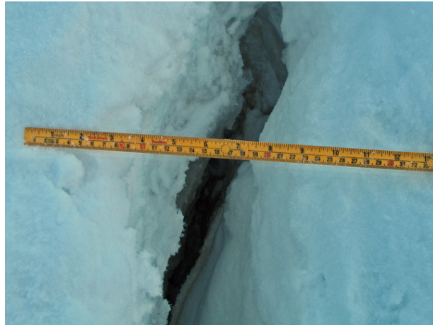
Figure B.58: Crack 1 opening at high tide (10-20 cm) – 22 February 2007 (week 8)
