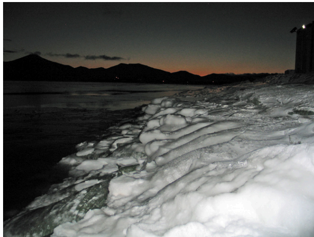
Figure B.10: Bags at the tip of the breakwater, looking toward west, sea height = -0.5 m – 1 November 2006 (week 44)
