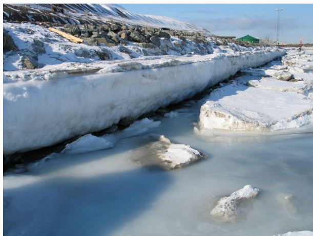
Figure 2.4: Ice foot on a steep slope in the winter. Port of Longyearbyen – 27 April 2005
