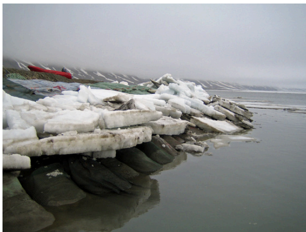
Figure B.116: Ice pile-up at the tip of the breakwater, sea height = -1.0 m – 19 June 2007 (week 25)
