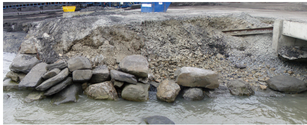
Figure C.1: Shore protection attempt with low-quality, local rocks at Kapp Amsterdam – 17 July 2007
