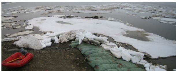
Figure B.115: Ice pile-up in the east corner of the breakwater, sea height = -0.8 m – 19 June 2007 (week 25)
