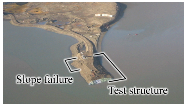
Figure 4.4: Aerial view of the breakwater – 30 August 2006
