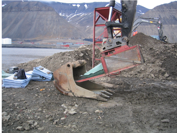
Figure C.11: Transferring a bag from the box to the bucket
