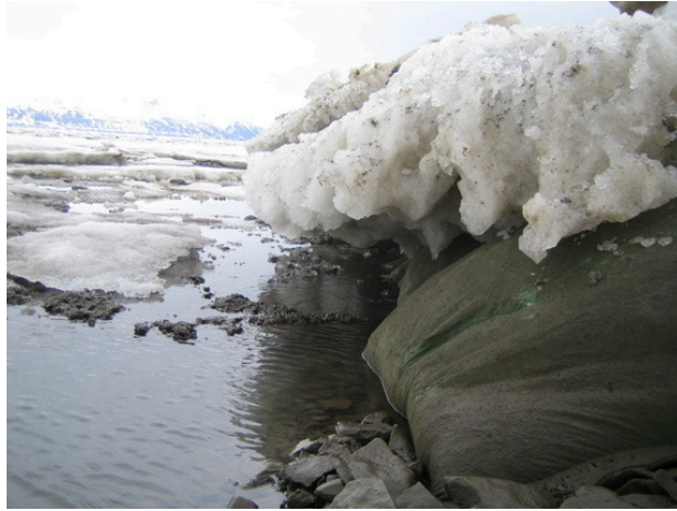
Figure B.103: Bags exposure following the melting of the ice foot, eastern part of the breakwater tip, sea height = -0.9 m – 16 June 2007 (week 24)
