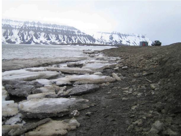
Figure B.99: Stranded ice blocks on the east side of the breakwater, sea height = -0.6 m – 16 June 2007 (week 24)
