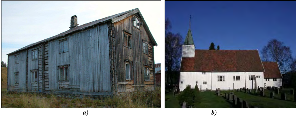
Figure 2.4. a) Old farm house in Bardu with pine heartwood cladding exceeding one hundred years, the different climate exposure is seen in its colours. b) The church in Søgne, sanctified in 1640, still with its original cladding.
