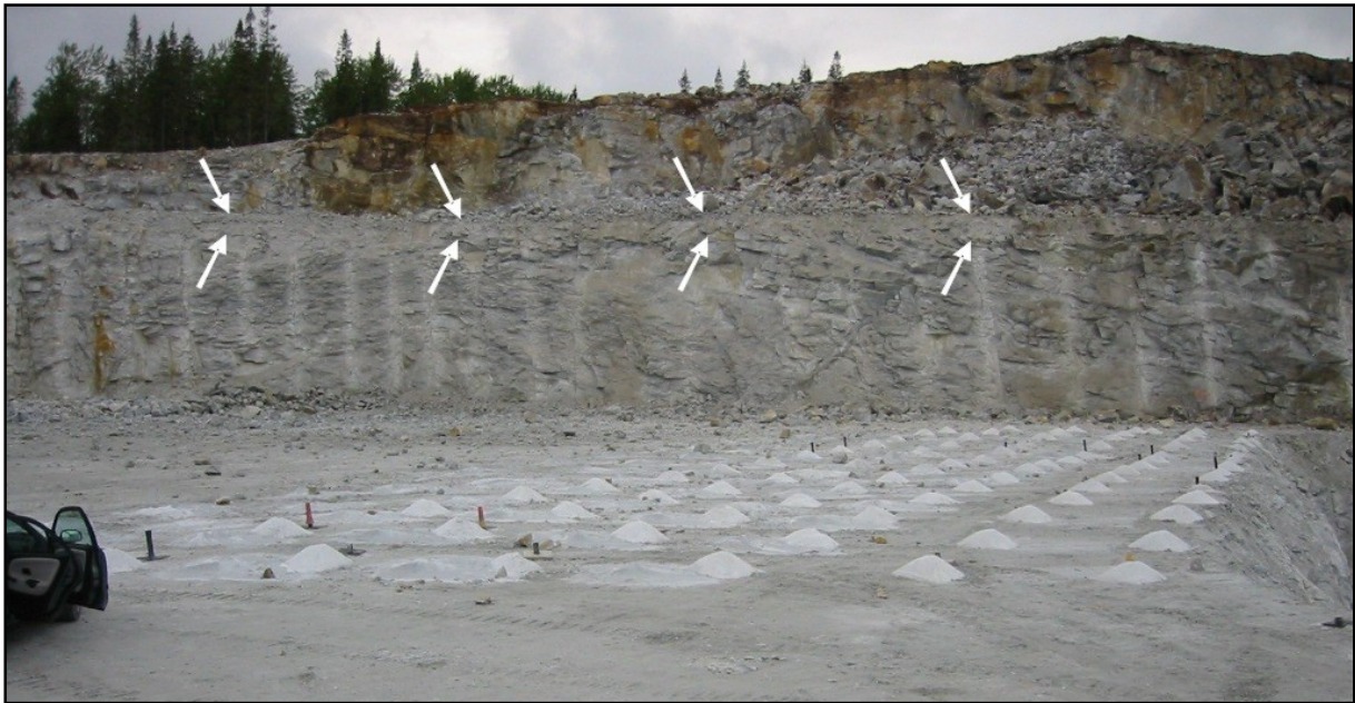
Figure 1 Blast ready for charging at Brønnøy Limestone Quarry, Norway. Holes drilled through the rock debris. Even bench floor conditions. The arrows point out the rock debris for the overlaying benching level. Photo: Vegard Olsen.
