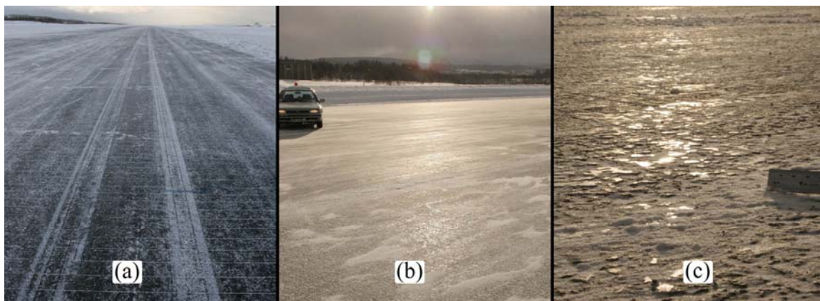
Figure 3-14. (a) Tracks of compacted snow resulted in spatial variability of the contamination. (b) The thin ice cover is visible by the reflected sunlight. (c) The asphalt texture is still visible and the top of the aggregates is covered with a thin layer of ice.
