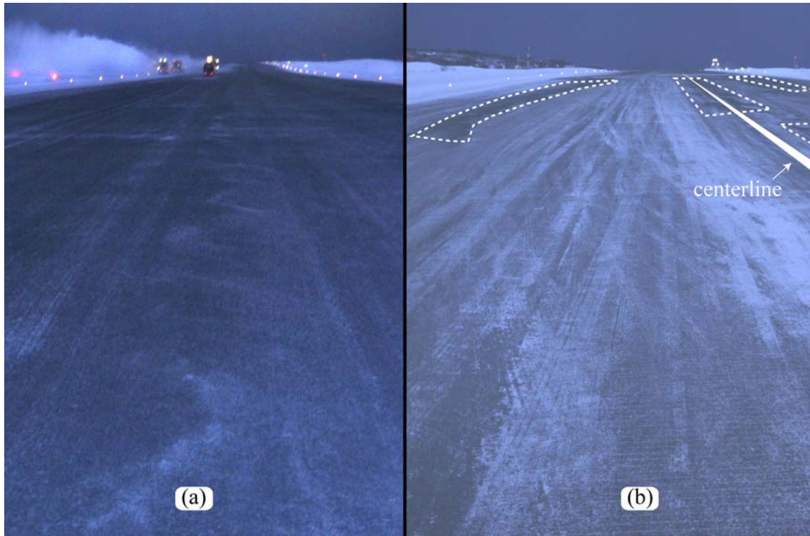
Figure 3-6. The runway surface conditions on January 26 (a) during friction measurements at 08:00 and (b) 11 minutes later, after three aircraft movements. The sand, initially uniformly distributed has been blown to the sides and towards the centreline. The regions with sand are indicated by dashed lines.
