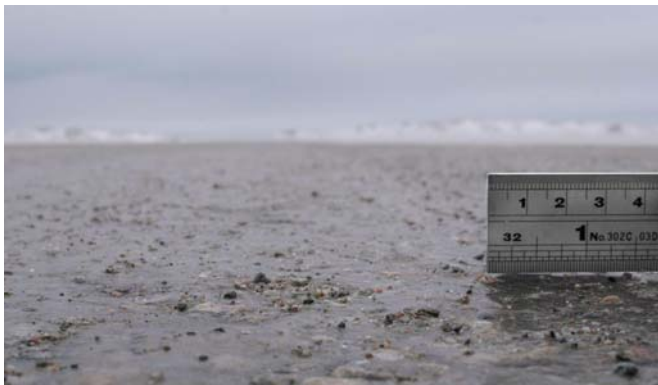
Figure 9-5. Example of an iced runway that is regularly treated with freeze bonded sand, four days after the last application.
