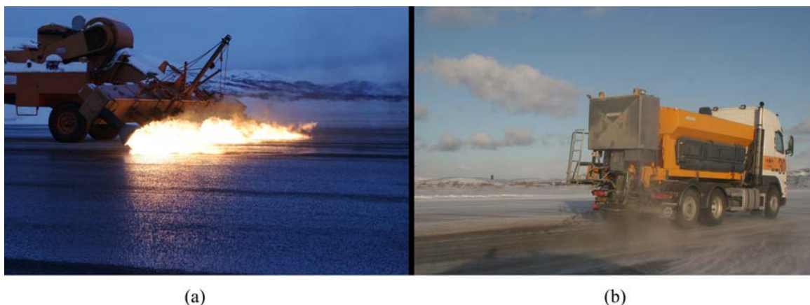
Figure 9-1. Traditional and modern methods of freeze bonded sanding. (a) The iced pavement is heated with open flames prior to the sanding operation. (b) A modern sand spreader that pre-wet the sand with hot water.
