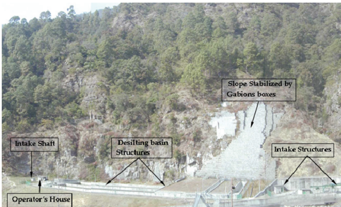
Fig. 1.2 Important structures built at the base of the slope (KHP) (Aryal & Sandven 2005)
