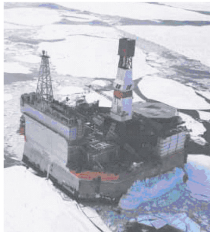
Figure 3.35. The caisson structure Molikpaq under ice actions at Sakhalin II deployment in the Sea of Okhotsk, Russia.
