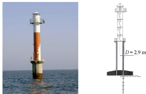
Figure 3.9. Vallinsgrund lighthouse ( D = 2.9 m) (photo: Swedish Maritime Administration).
