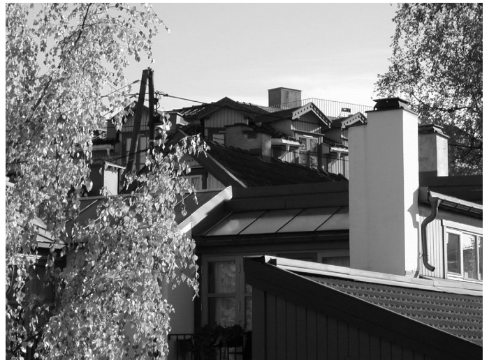
Figure 2. The traditional type of roof for dwellings in Norway are ventilated and insulated pitched roofs (photo: K.R. Lisø).
