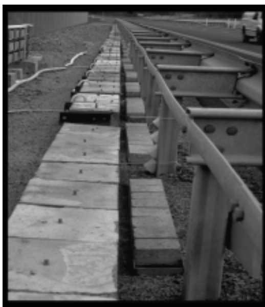
Figure 5.2.1 : Location of 15 x 15 x 7 cm 3 samples at the site. Also larger samples for other purposes like corrosion measurements etc. are located here. Front side faces traffic and is directed towards south. From [U 1999c].
