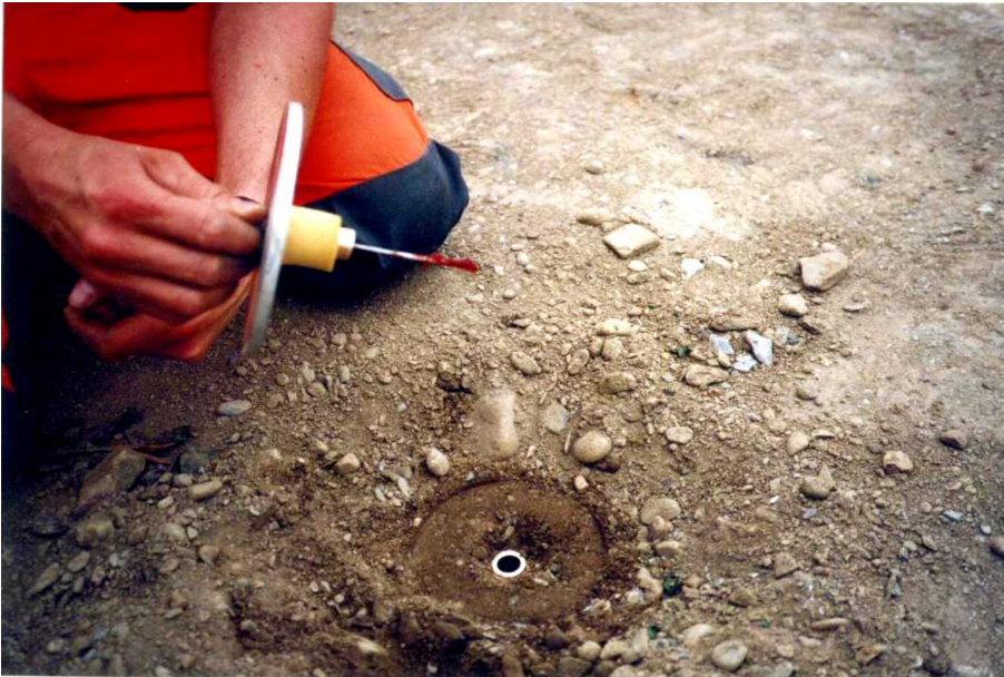
Figure 4-23: Installation of a VDT in the subbase layer
