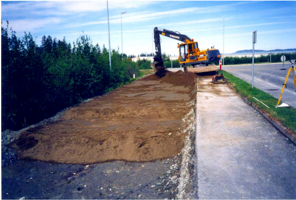
Figure 4-5: Placement of the sand layer
