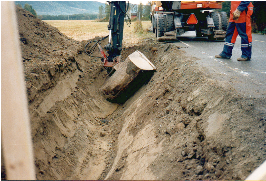
Figure 3-17: Excavation from the side of the road at Fv 462
