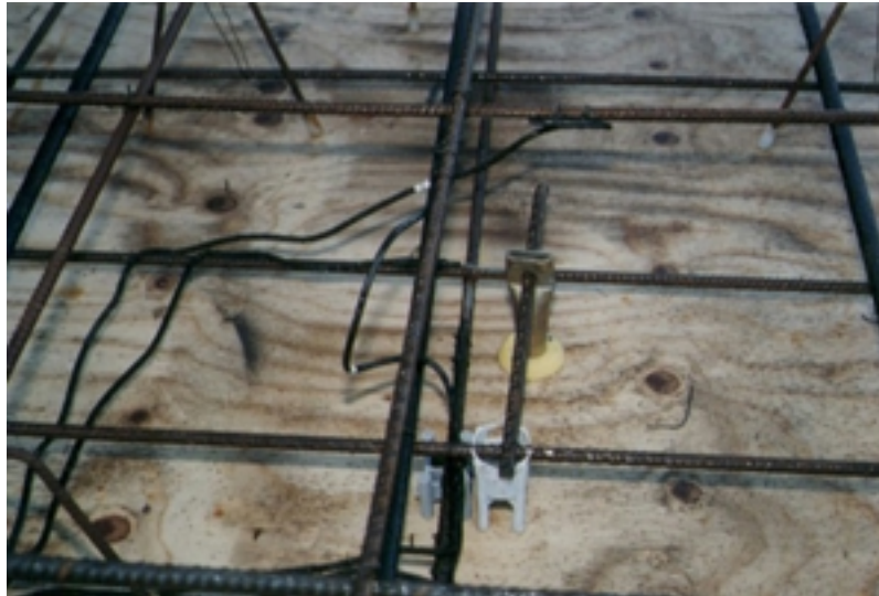
Strain gauges and measure point.
