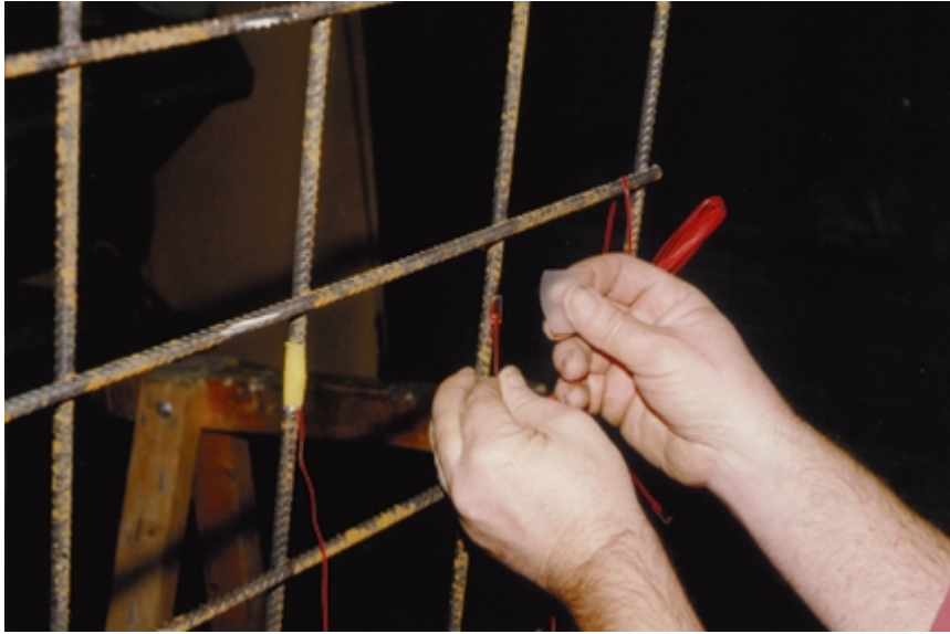
Strain gauge glued at reinforcement. Figure 6.20
