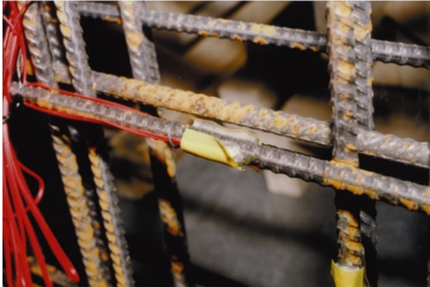
Strain gauge at both sides of reinforcement.
