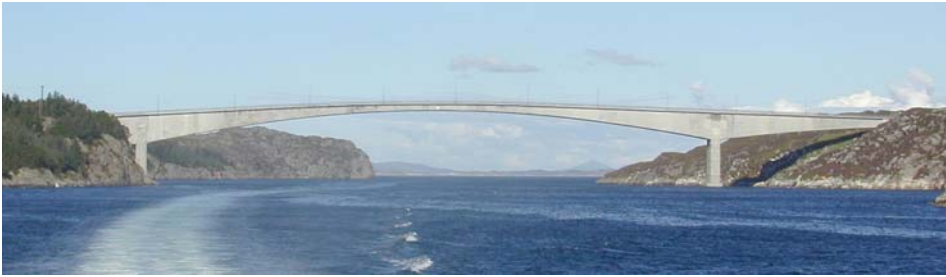
Figure 2.2 Stolma Bridge, world record in free cantilevering
