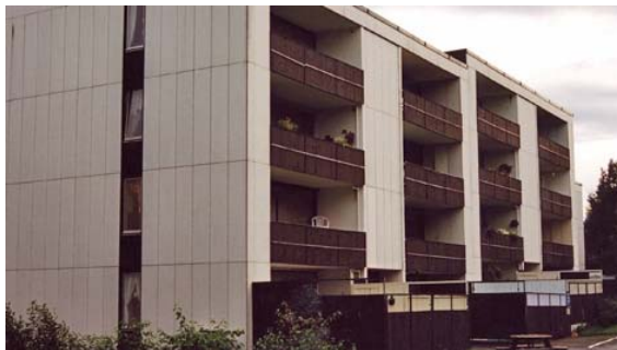
Figure 1: Photo, Blocks of flats on Kolstadflata, case A.
