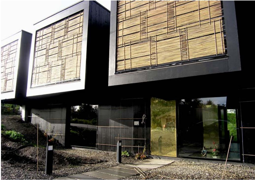
Entrance elevation with front door covered in brass (photo: Bård Helland).
