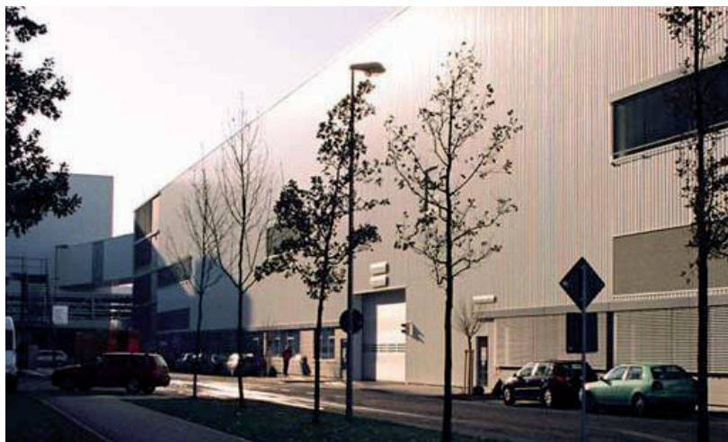
Figure 7-20. Photo of production hall exterior (Courtesy: Obermeyer Planen + Beraten).
