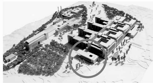
Figure 2. The AHUS project and the front building (Illustration: C.F. Møller Architects).
