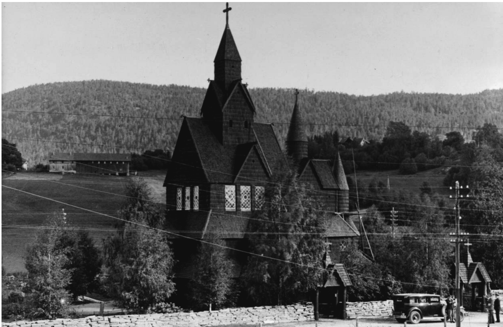
Figure 5-6: Heddal stave church, drawing by P. Hansen August 1851 (top) of the newly restored church, and photograph by Domenico Erdmann from 1934 or 1936. P. Hansen's drawing of the newly restored church was presented in Fortidsminneforeningen's annual publication of 1851. (Fortidsminneforeningen, Domenico Erdmann©Riksantikvaren, both Riksantikvaren archive)
