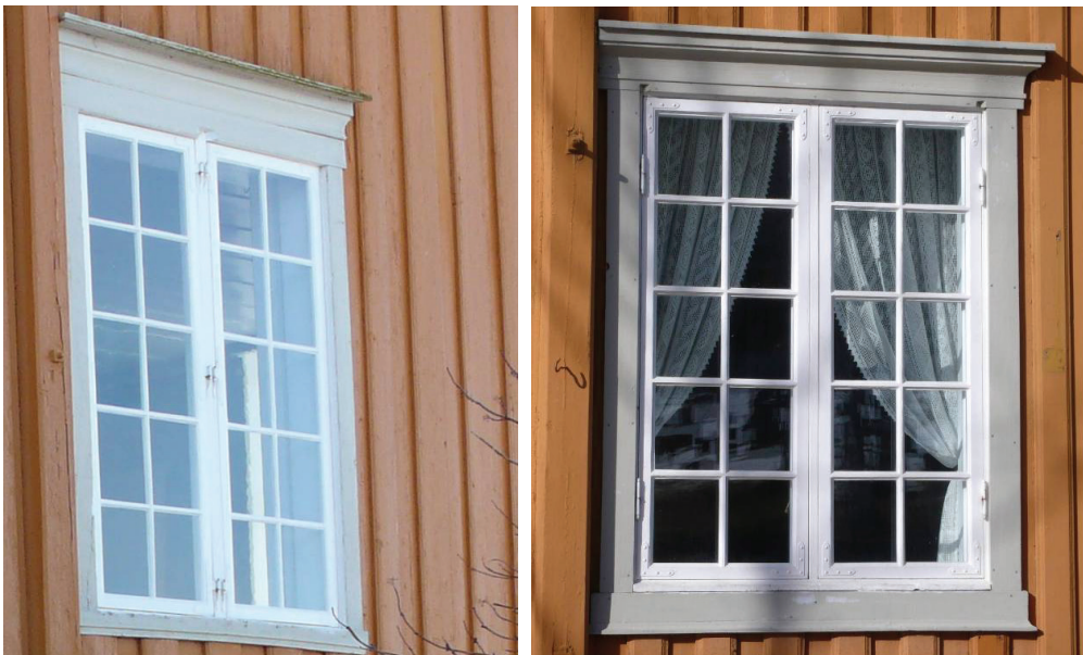
Figure 36-37: 18 th century window in Prestegårdslåna in the west end gable (left), moved here from Herrestuen and reused in " Almuestuen " in connection with the modernization in 1877 and the only larger window from before 1877 is preserved in the building. Double glazed ( koble ) window from the 1929 restoration (right) designed by architect Roar Tønseth, likely modelled after " Almuestuen "'s. (Photographs MB 2009)
