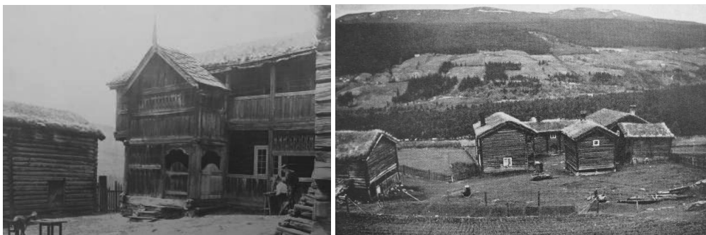
Figure 1-2: "Heidal Harildstad Søndre Foto Schirmer". Schirmer students at Harildstad Søre (left), and Søndre Harildstad presented as an example of a repaired listed building in an article by Harry Fett and Halvor Vreim (right), Fortidsvern og ungdomsarbeid from 1941 with the caption: "In this farmyard all buildings are repaired. New foundations and to some extent basements. Walls and roofs repaired." 3 (Photographs unknown©Riksantikvaren)
