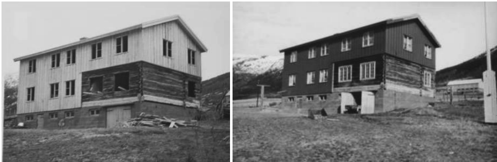
Figure 13-14: Krogstad in 1958. The new house envelopes the section from 1811, still under construction (left) and finished with windows and paint and a car in the new garage (right). Vreim initially rejected the plans to place the garage under the 1811 rooms; he also wanted the 1811 section left exposed, but it was clad shortly after the house was finished. His request that the whole house was given small-paned type casement windows was also ignored; the owner wanted a more modern window type and Vreim's preferred type ended up being used for the 1811-section only. (Photographs: Halvor Vreim ©Riksantikvaren)
