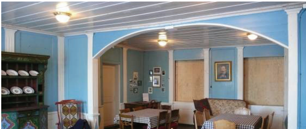
Figure 31: Hovdenstova where two rooms were joined during Vicar Anders Hovden's residency between 1910 and 1920. In 1929 the southern wall was fitted with new doors to the veranda which were disguised as windows to complete the image of a dadoed wall. The bottom panels can be removed, and the open space behind them filled with heat insulation material. (Photograph MB 2005)
