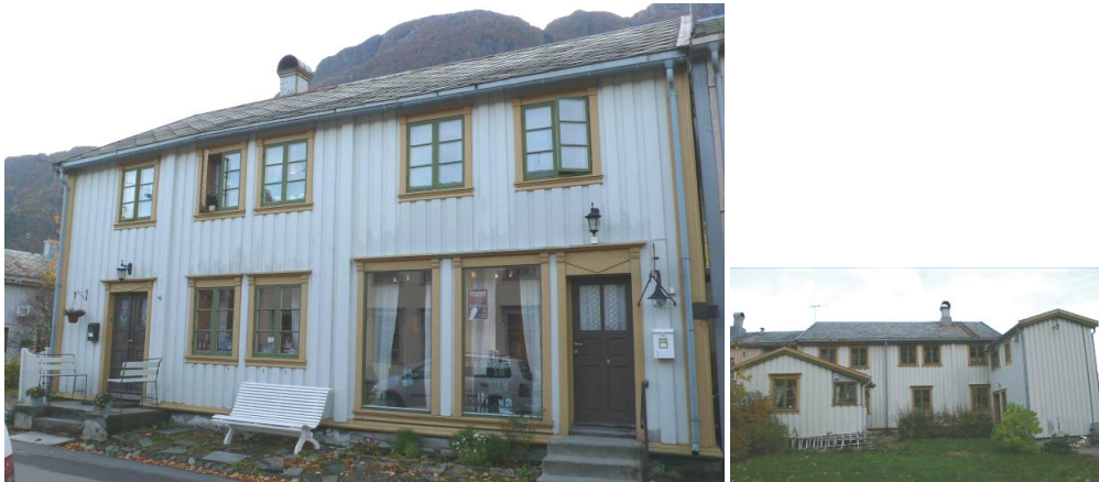
Figure 11-12: Sjøgata 41 street façade (left) and backyard façade (right). (Photograph MB 2007)
