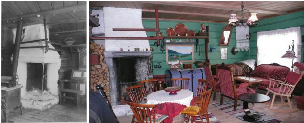
Figure 19-20. The old fireplace in the Krogstad stugu (left) and the new fireplace as it was reconstructed in 1956 (right). Vreim's specifications were: "Even if the new chimney is placed behind the fireplace, the fireplaces must not be altered upon reconstruction. This also relates to the character of the rendering of the overmantel. As much as possible of the old stone is to be re-used." 121 The photo of the room before the relocation shows that an iron stove had been fitted by the old open fireplace, with a hazardous stack penetrating the wooden ceiling. These furnishings were not included when the room was reconstructed; it was restored to a previous phase. In the right hand corner can be glimpsed the bed fixed to the wall, which was noted missing by Vreim upon his first visit, and reconstructed after the building was moved. Under this room the owner built his basement garage, with the entrance gates directly under the window. (Photographs: Halvor Vreim ©Riksantikvaren, and MB 2008)
