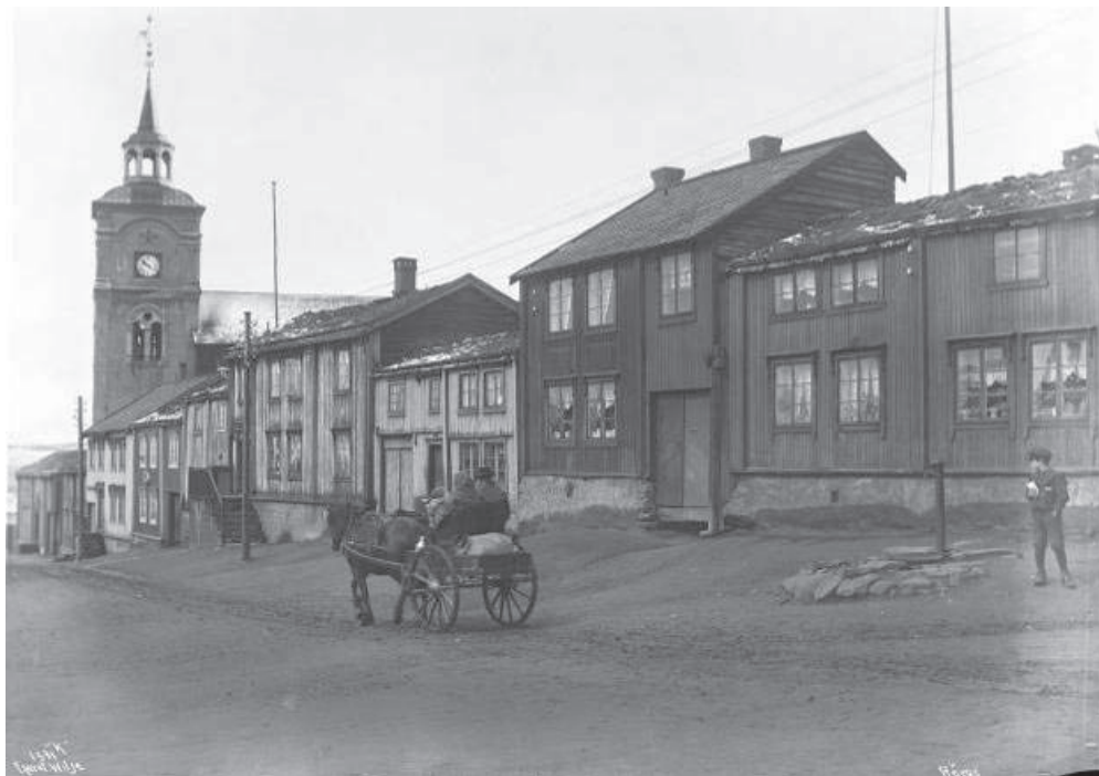
Figure 12-13. Sohlbergrekka in 1903 (top) and 1914 (bottom). The building to the far right in all photographs is Kjerkgata 60. (Photograph Anders Beer Wilse 1903 ©Norsk Folkemuseum, reproduced with permission. )
