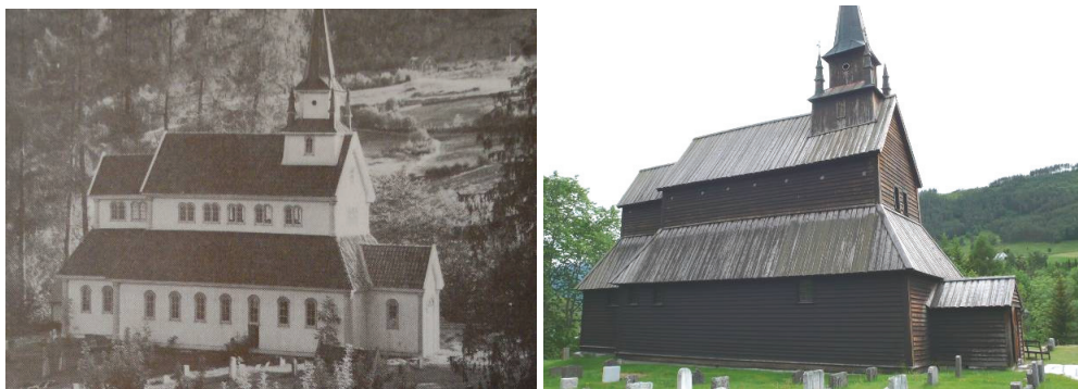
Figure 37-38: Kaupanger stave church after Stockfleth’s modernization in 1862 (left); in 2010 with the exterior it obtained from Kristian Bjerknæs’ restoration in 1952-64 (right). Bjerknæs based the new exterior on paintings and drawings from the early 19 th century which showed that the church had been clad with wooden planks. The exterior work was carried out in 1964 in the second phase of the restoration.
