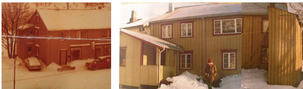
Figure 15-16: Sjøgata 41 in 1977, street and courtyard façades as they were in the 1960s and 1970s. The building still had some of its older windows intact; in the right hand photo an upstairs window is slightly open, showing that it was hinged on the mullion. In the photo: architect Dag Nilsen. (Vefsn municipal building archive)
