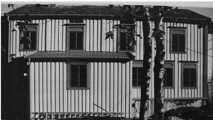
Figure 55-57: Sjøgata 37, backyard façade before regeneration (top); backyard façade after the secondary addition was removed (middle); new backyard addition in place (bottom). (Photographs: Dag Nilsen, Dag Nilsen private archive)
