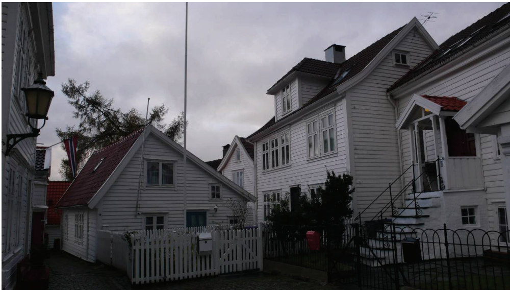
Figure 52: Rosesmuggrenden 9 (left), 7 (centre right) and Garmannsgate 8 (right). Rosesmuggrenden 7 underwent a comprehensive rehabilitation in 1987 which involved a complete renewal of the interior and transformed the building from a 19 th century apartment building to a two-apartment building conforming to 1987 building standards. The red tile roof was replaced with a black concrete tiles of the brand “H-panne”. The main timber construction was preserved. Façade cladding and mouldings were renewed. The original windows had already been replaced with modified copies in 1978. (Photograph MB 2005)
