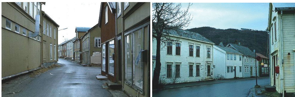
Figure 5-6: Boarded up windows and peeling paint: Sjøgata in 1978. (Photograph Håvard Dahl Bratrein 1978 ©2009 Tromsø Museum, UiT)
