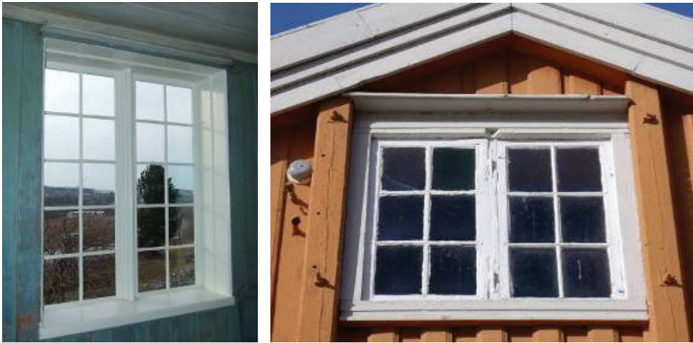
Figure 34-35: Only two 17 th century windows are preserved in Prestegårdslåna's façades. The fire insurance valuation from 1868 described six different sizes of windows, including these two. The larger window (left) which has 20 panes, is placed in the west end gable wall, in Borgestuen . It was moved from Herrestuen and reused here in the 1878 modernization. Roar Tønseth used this window as a prototype for his restoration design. The smaller window has 12 panes and is placed in the loft section of the east end gable. Both windows are hinged on the mullion. The remaining windows in Prestegårdslåna are from 1878 or the 1929 restoration. (Photographs Kristine Kaasa Moe; MB 2009)
