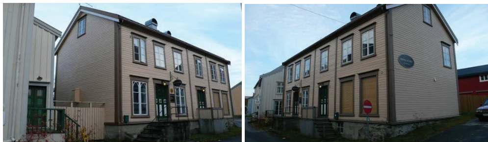
Figure 31-32: Sjøgata 26 street façade looking in the southern (left) and northern direction (right). (Photograph MB 2007)
