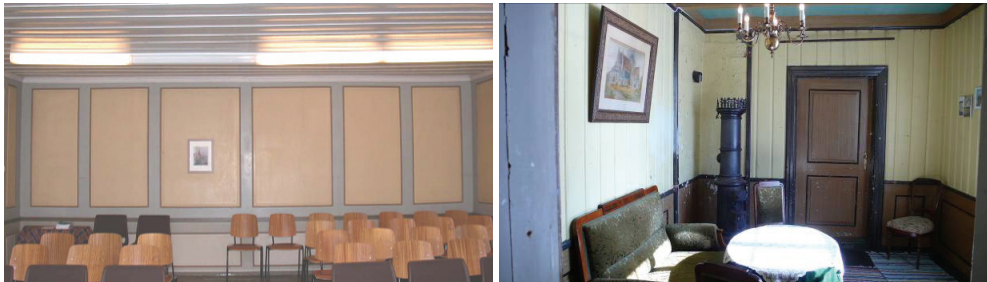
Figure 32-33. Herrestuen (left) was the congregation's responsibility until 1908. Originally with exposed timber walls, the room was frequently described as draughty. Panels were mounted during the first half of the 19 th century, and the ceiling in 1877-78 when the whole building was modernized. The room was proposed to be divided but architect Tønseth argued against this. It was last painted in 1929 for Tønseth's restoration. 252 The bishop's chamber (right) was the shared responsibility of the vicar and the congregation during the 18 th and early 19 th century. Over time this room has had the function of bedroom, office, sitting room and kitchen. In 1922 Tønseth proposed to fit the doors leading onto the terrace here, but these plans were abandoned. (Photographs MBY 2005)
