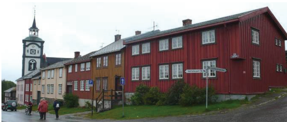
Figure 1-2. Aerial view of Røros 2003 (left). Røros historic town has a baroque plan in which a larger street has a faux perspective with the Copper Mine Director's house as a monumental backdrop in the widest section. The case study area Sohlbergrekka (right) is found in the upper section of the smaller street, Kjerkgata (“Church Street”) or Litj-gata (“Little Street”). As in Røros, wood also constitutes the main building material in many of the country's other historic town cores and hamlets, as well as in rural architecture. As a historic wooden townscape, Røros has both unique and representative values. (Photograph Dag Nilsen; MB 2007)
