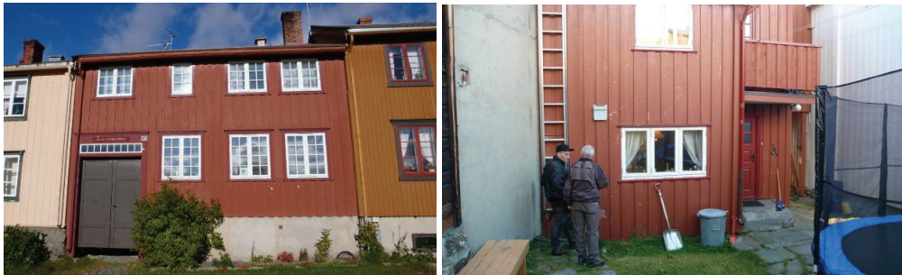
Figure 36-37: Kjerkgata 56, street façade (left) and backyard (right). (Photographs MB 2007)
