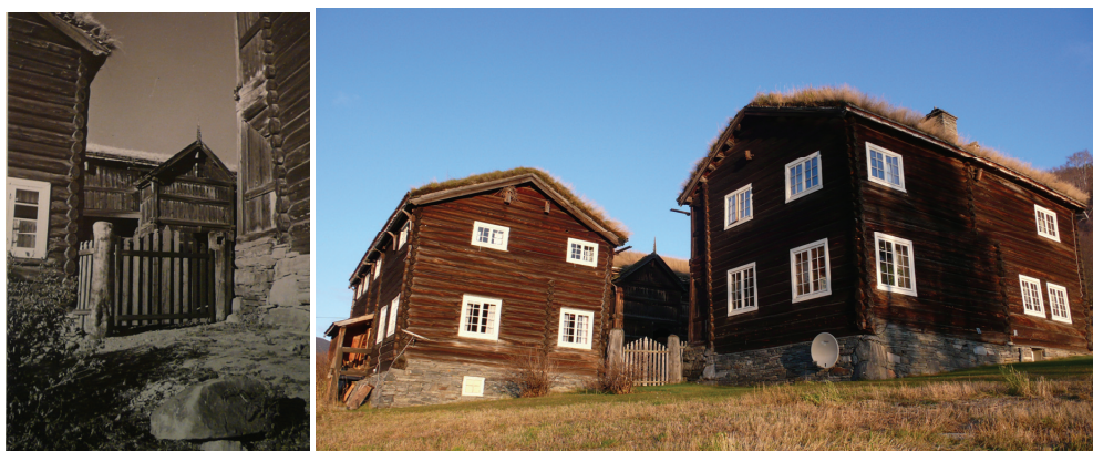
Figure 54-55: The farmyard in 1938 (left) and 2008 (right) with Nedre Stugu on the left hand side, the Nordre Stugu gallery centre and Søre Stugu to the right. The upstairs windows in Nedre Stugu were fitted after 1946. Den Antikvariske Byggningsnemnd was consulted on the matter. (Photograph Halvor Vreim 1938 ©Riksantikvaren and MB 2008)
