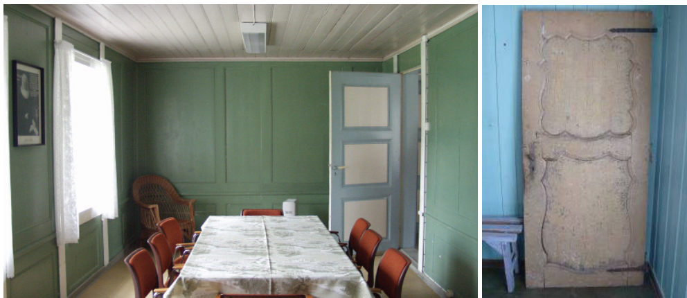
Figure 12-13. Lystersalen (left) in the oldest part of Prestegårdslåna, named after the vicar Christen Lyster who had this section built in the 1720s. Examination of the wall panels revealed their original colour as dark green 111 ; an incision in the ceiling boards indicated a previous staircase at the far end of the room. This may have been removed in 1877, when the room according to written sources “extended”. The door (right) is the larger of two early 18 th century doors found in the west end. Its likely origin is the oldest section of the building, maybe between Hovdenstova and Bispekabinettet . It was temporarily reused as an exterior door to a utilities building. 112 (Photograph NIKU 2003; MB 2009)
