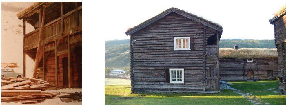
Figure 58-59. “Søre Harildstad Sørstua under restoration March 1976” (left), and in 2008 (right). The ground floors of Søre Stugu were replaced after a fungal attack in the northern section of the house. The gallery was partly dismantled and the sill replaced. The sill log was replaced in 1976. The surface of the new log has surface tracing of axe work and seems to have been tinted to blend in with the old wood. The windows were renewed in 1982. (Photographs unknown ©Riksantikvaren and MB 2008)
