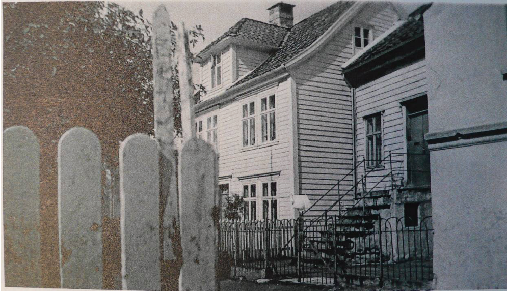
Figure 51: Rosesmuggrenden 7 (left) and Garmannsgate 8 (right) “Rosesmuggrenden sept. 1960”. (Photograph: Sollied, Rosesmuggrenden Velforening, Gamle Bergen Museum archive)
