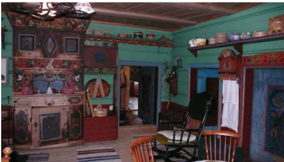
Figure 17-18. Interior of the stugu with cupboard, main entrance and door to the smaller chamber before (top) and after reconstruction. This section of the house was completely disassembled, rebuilt with laftevatt (fabric chinking) instead of moss between the timber logs. The interior was restored by a local painter on the instructions of Riksantikvaren 's restoration assistant Ola Quale. The wall paint, green, is from the late 1950s, based on the original colour. The doors and fixed furniture do not seem to have been touched. The rooms are an integral part of the house in 2008, but not in daily use. Right: (right). Photo Halvor Vreim ©Riksantikvaren (Archive B123). Photo MB 2008
