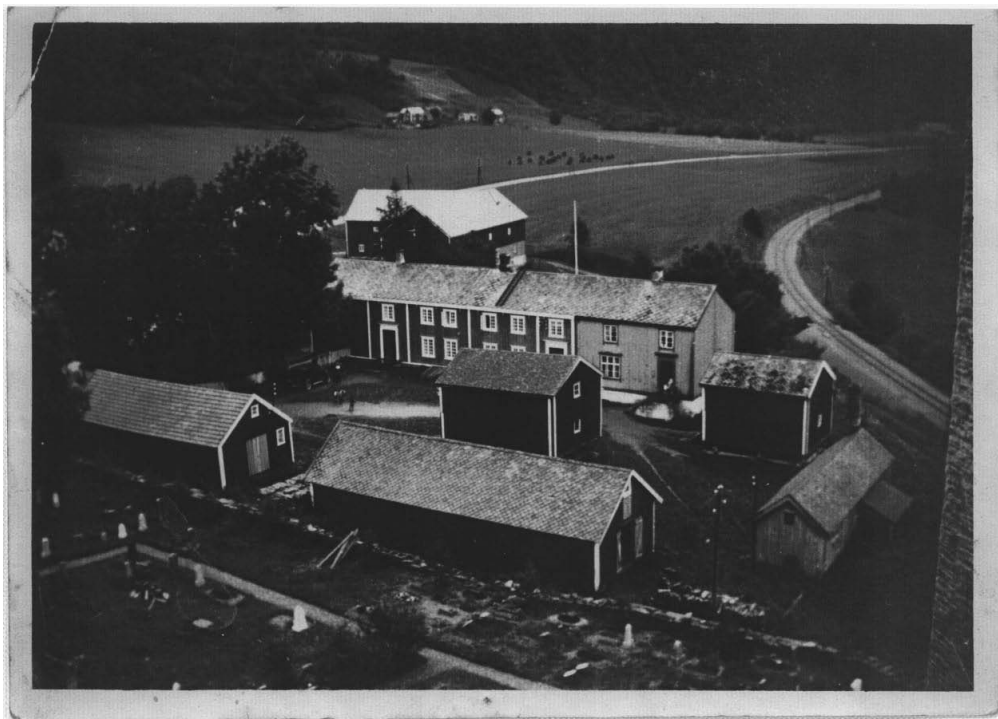
Figure 39: The north façade of Prestegårdslåna and the old farmyard photographed from the tower of Melhus church in 1937/38. The restored section was painted red, while the west end section which here is the right hand side of the building remained yellow, and retained its windows from 1877. The utilities buildings; wagon shed, wood shed ( rulle og -vedbu ), two storage buildings and drying house; were demolished after Melhus municipality took ownership of the vicarage in 1959. Riksantikvaren protested, but arguments that the buildings were too costly to maintain won. The new utilities building, in the background, replaced the older barn, cowshed and stable. In 1948 a new dwelling for the tenant farmer was built south of the utilities building.
