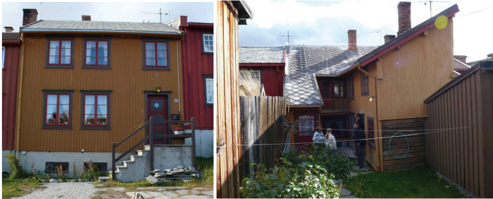
Figure 51-52: Kjerkgata 58 street façade (left) and courtyard façade (right). (Photograph MB 2007)
