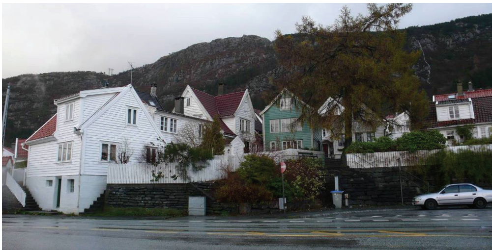
Figure 42. Rosesmuggrenden. Fjæregrenden 18 to the left. Its neighbour Fjæregrenden 20 was demolished with the extension of Sjøgate, leaving the west façade exposed to the street. New tall concrete foundations and steps were constructed to negotiate the difference in height. The arched dormer was reconstructed, the Empire Style windows replaced with a type associated with functionalism. All these alterations were performed before 1953, and before the municipal guidelines of the “conservation plan” were adopted. (Photograph MB 2005).
