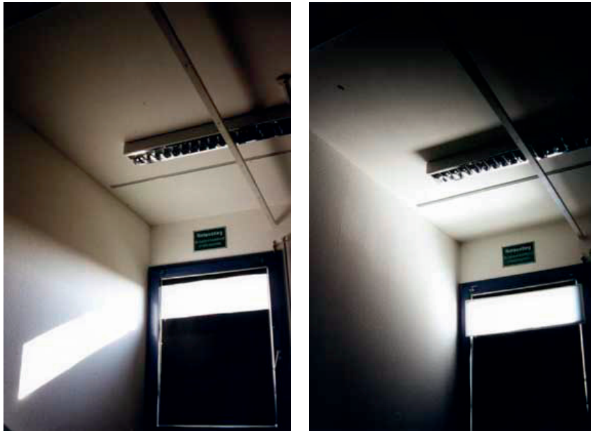
Figure 3-19 Illustration of light distribution in a sidelighted space without (left) and with (right) sun-directing glass in the clerestory portion of the window opening. Pictures reprinted from the (former) website of the company LIFLITE GmbH.
