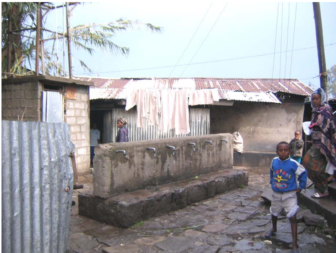
Fig. 5.11: In-situ maintained house
