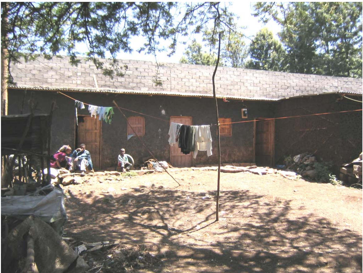
Fig. 7.8: Newly constructed houses
