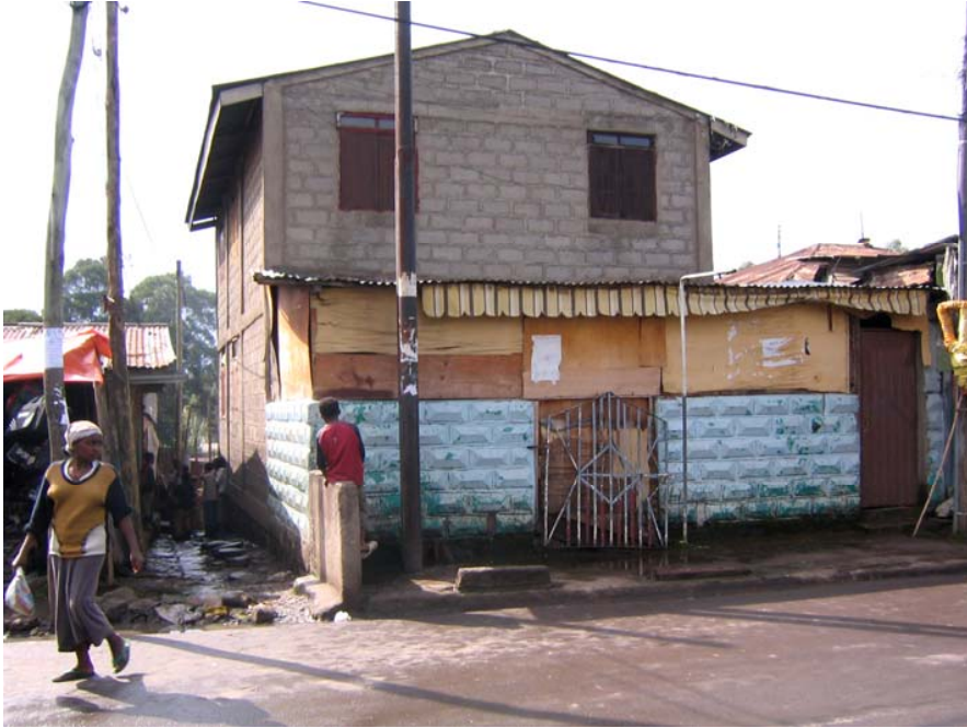
Fig. 5.13: Encroachment towards street
