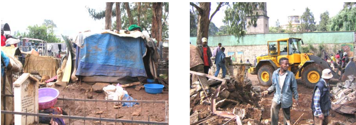
Fig. 4.16: The squatters and the cemetery being bulldozed
