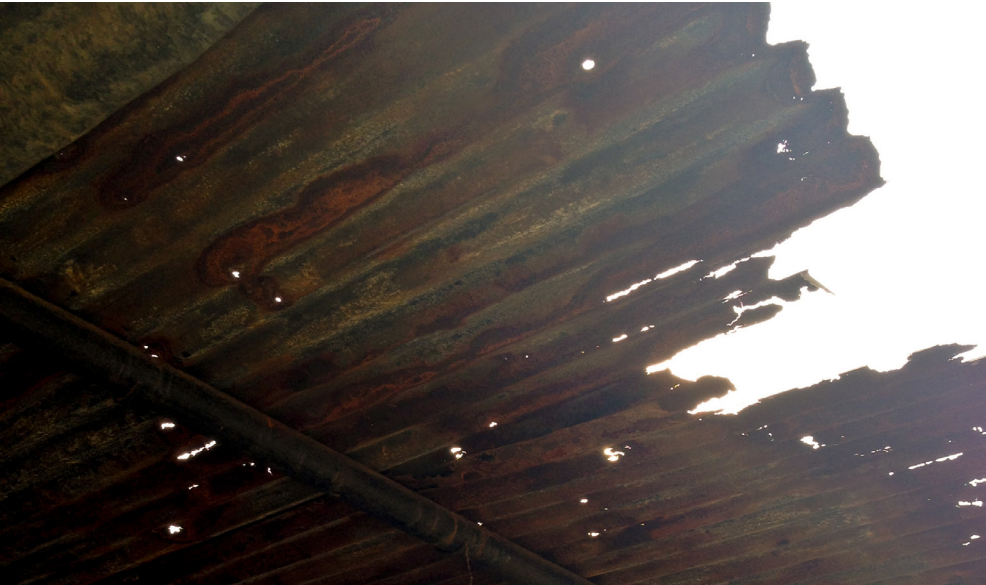
When constructing the roof in the community center the NGO introduced a recycled plastic material. Today, the roof has started to melt.
