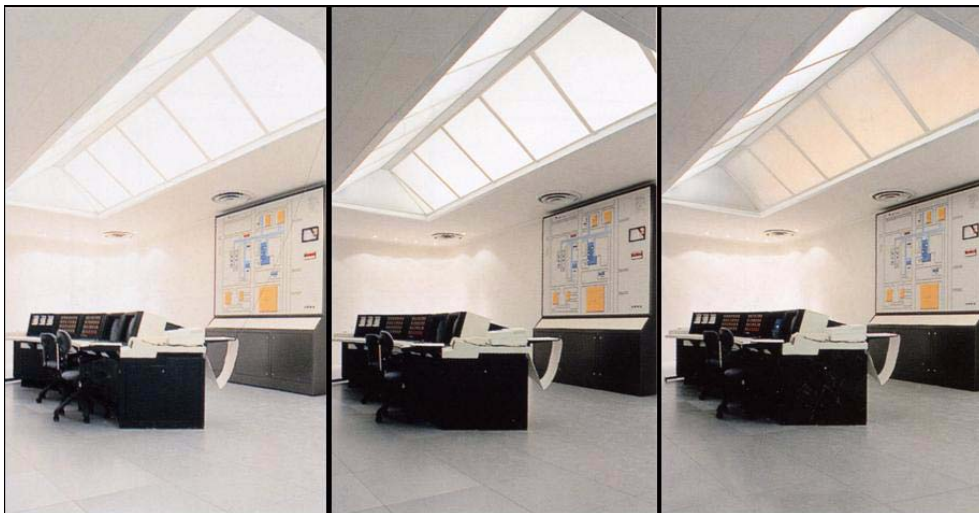
Figure 5-36: The SIVRA artificial skylights, installed in a control room, varying in colour and intensity during the course of time.
