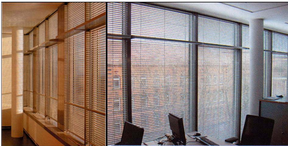
Figure 5-61: The PRO-day facade balancing glare protection, daylighting and visual contact.
