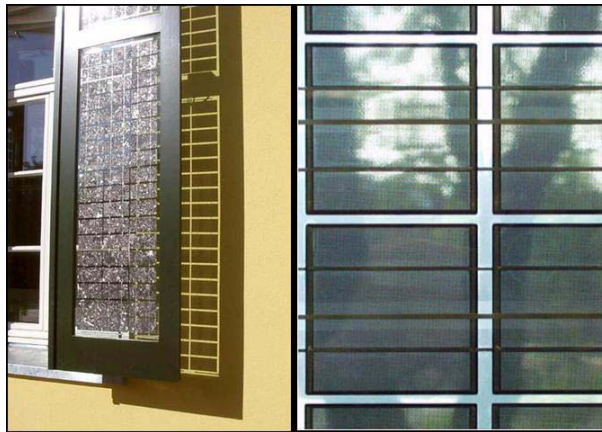
Figure 5-44: The semi-transparent shutters create shading patterns, while allowing for a distorted view to the outdoor environment.
