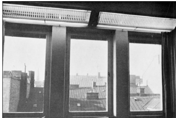
Figure 5-57: The Swedish variation of P.S.A.L.I. (Permanent Supplementary Artificial Lighting in Interiors), with artificial lighting installed directly above the windows.
