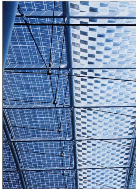
Figure 5-67: The ETFE foil cushions with closed and open solar shading (7 %, resp. 50 % visible light transmittance).
