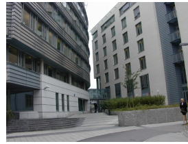
The bridge between E7 and E9
