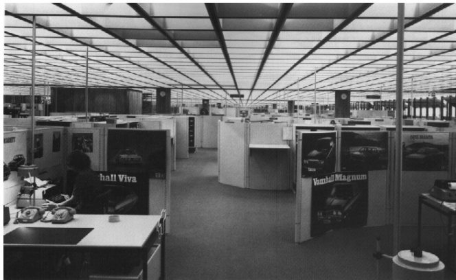
Topsikring, Ballerup. Denmark. 1974 (Flagstad & Laustsen, 1983)
