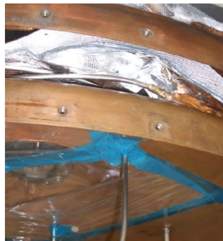
Fig.4.25. The pipes in the copper cover
