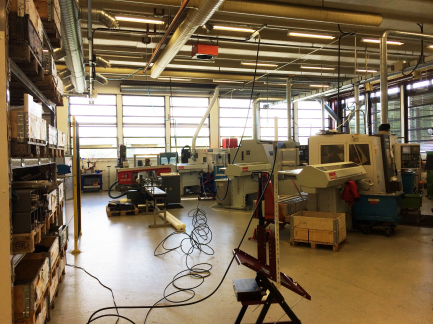
Fig. 3: Measured mechanical room.
