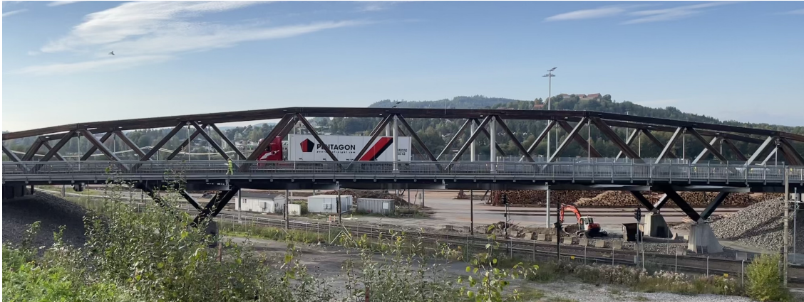
Figure 1: Norsenga Bridge viewed from the south
