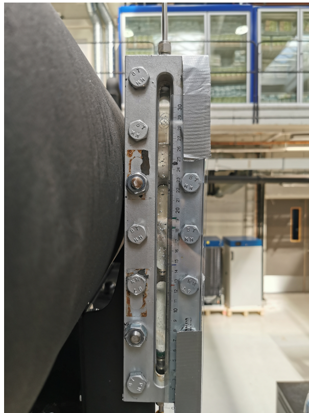
Figure 19: Sight glass to read the liquid level within the receiver tank
