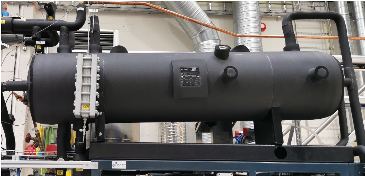
Figure 18: Gray water tank functioning as the receiver
