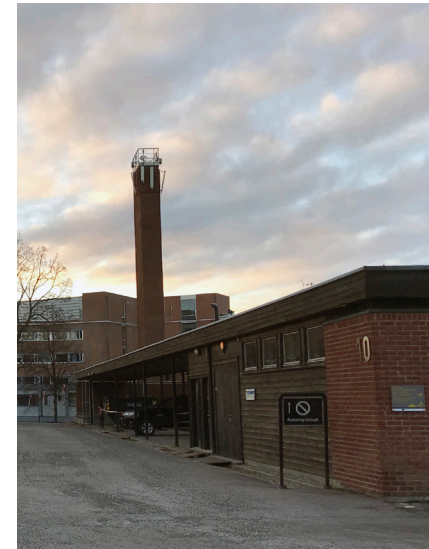
Boilerhouse and chimney. Photo taken by author.
