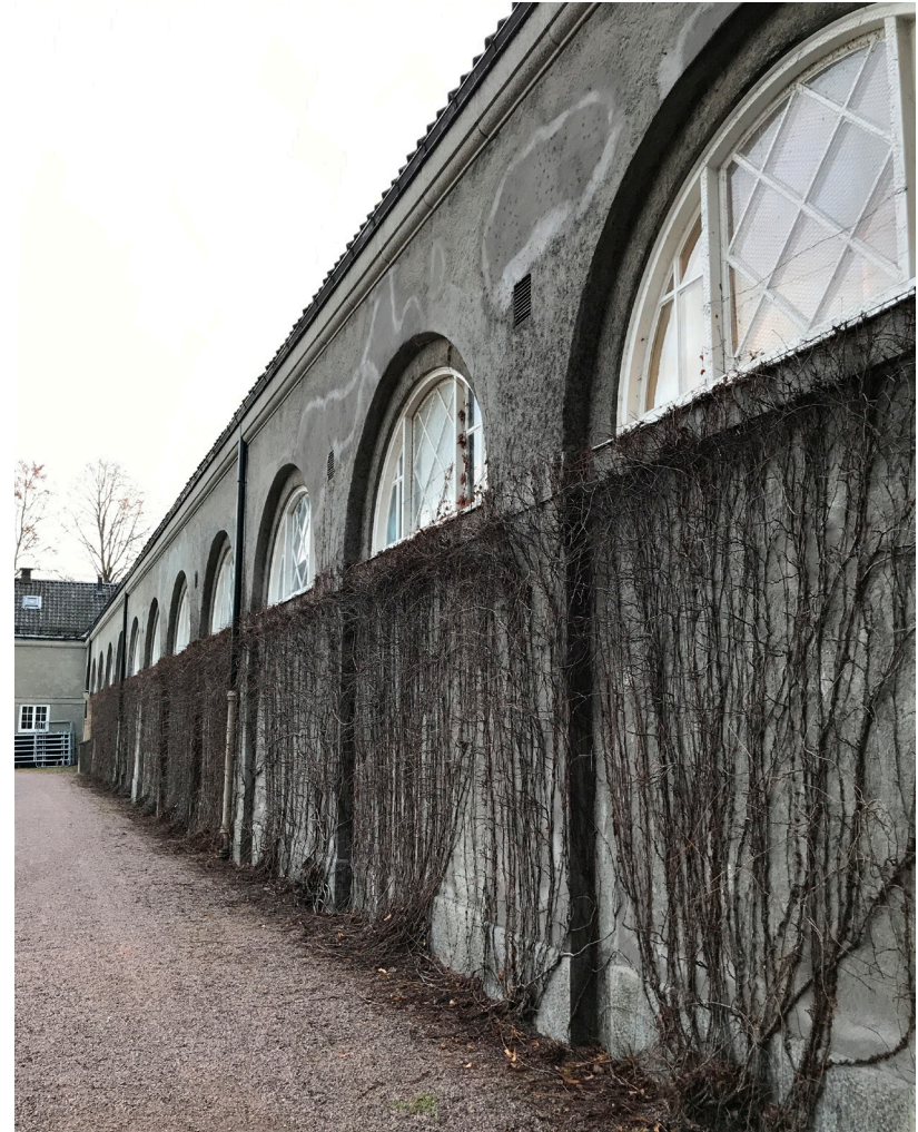
East Facade of Building 4, the Medical Clinic.
