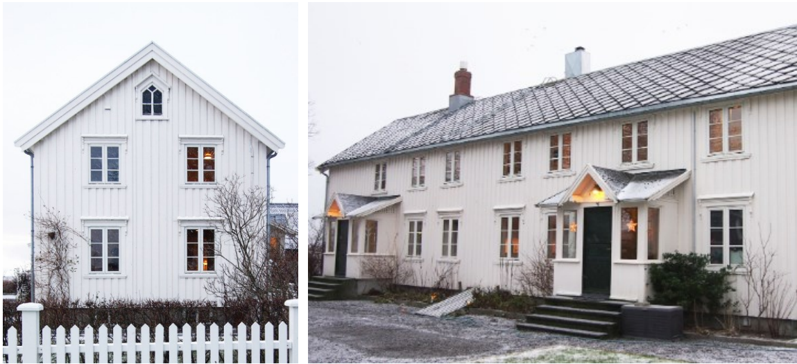
Figure 6.14: The east (left) and north (right) façade of Viken illustrating the current windows (Taftø Petersen & Johansen, 2015).
