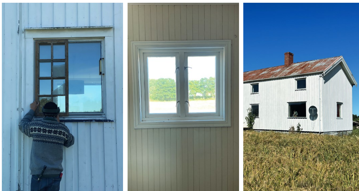
Figure 6.13: Left: Old slatted window found at the farm held over an awning window. Middle: two-section casement window. Right: Awning windows on the southwest and southeast façades. Photos: (Hesthol Løvik et al., 2022).
