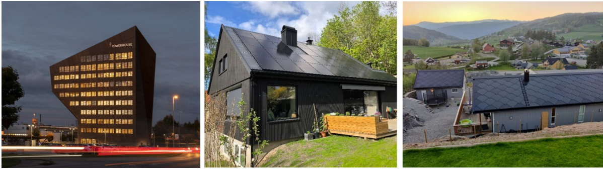
Figure 5.4: Powerhouse Telemark (left) (Powerhouse, n.d.). Two Norwegian houses with BIPV roofs (middle and right) (Bunkholt et al., 2021).
