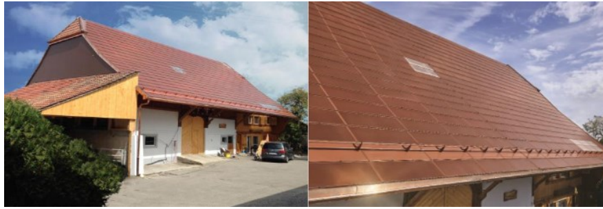
Figure 5.1: Rural farmhouse in Switzerland from 1859 with terracotta coloured BIPV (right picture). The left photo shows the building before the energy upgrade. Photos from (Polo López et al., 2020).
