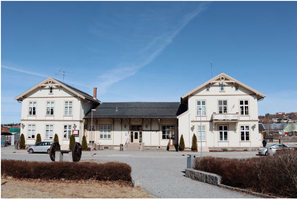
Figure 6.22: The central station building, author.
