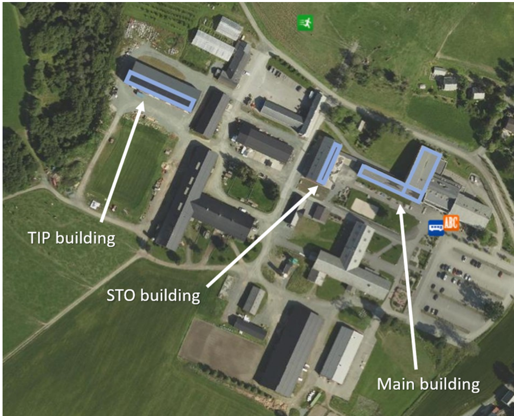
Figure 13: All existing rooftop PV installations at Skjetlein.
