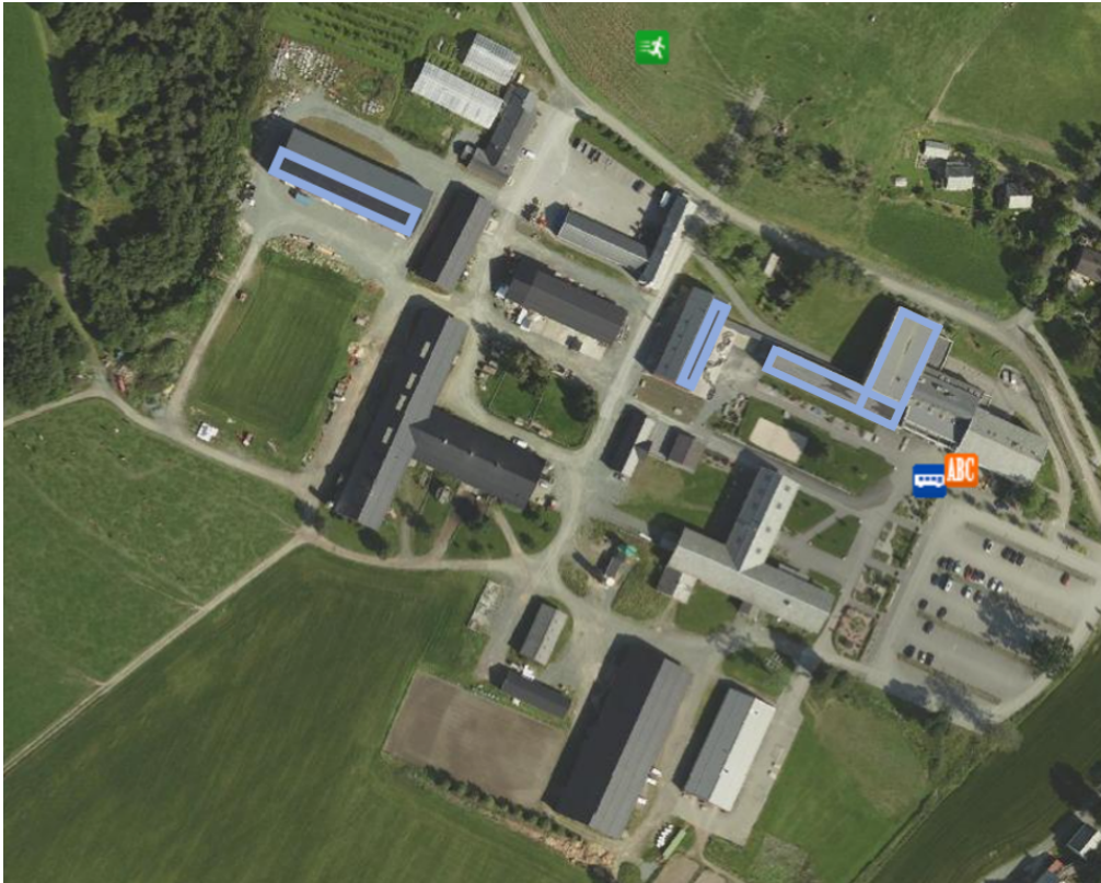
Figure 1: Aerial photography of Skjetlein High School showing the areas of existing rooftop PV installations marked in blue.
