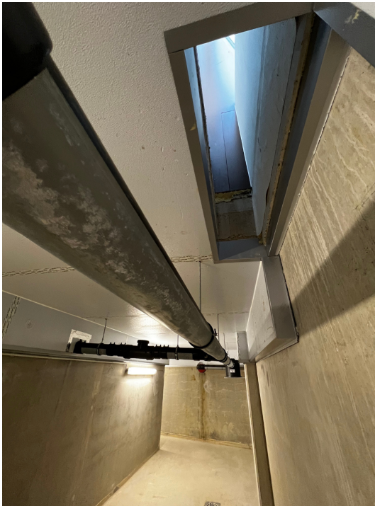
Figure 4.2.10: The outlet of the air flowing through labyrinth to the building, Photos taken by the author.
