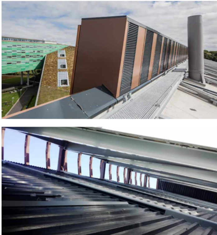
Figure 4.2.8: Solar chimney powers natural ventilation ( Energy Academy Europe , 2017)
