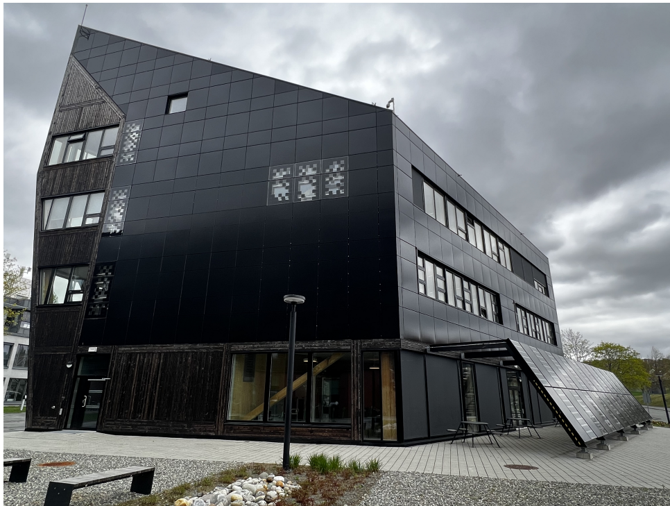
Figure 4.1.3: ZEB Laboratory, Southern and Western façade, Photo taken by the author.
