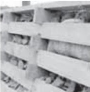
Figure 4. Crib wall
