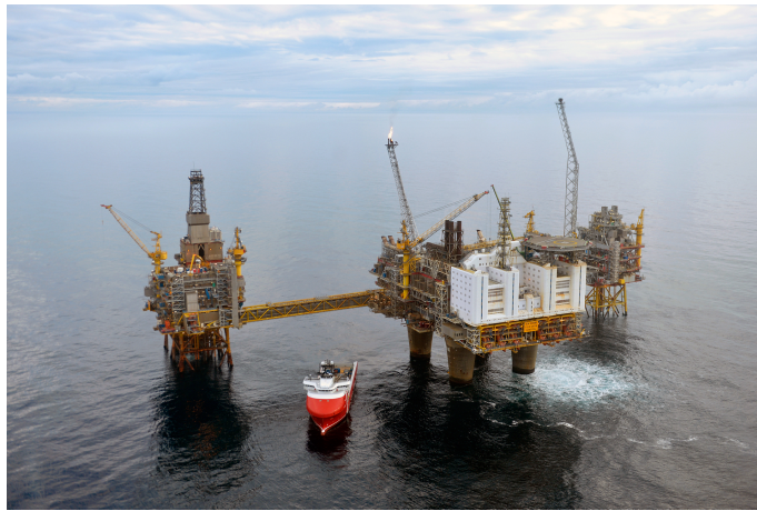
Figure 7: The Oseberg Field Centre. One of the platforms operated by Equinor, with a total of 21 oil and gas wells tied into the Field Center [4]. Courtesy Harald Pettersen – Equinor [5].
