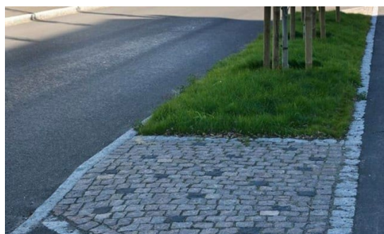
Figure 5-6: Second photo of street in Andenes showing green dividers and smooth transition. (Statens Vegvesen, u.d.)
