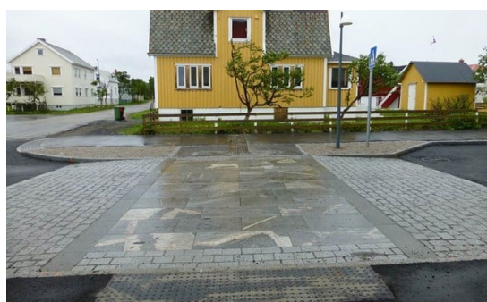
Figure 5-8: Fourth photo of street in Andenes showing ramps up to sidewalk-level by crosswalks. (Statens Vegvesen, u.d.)
