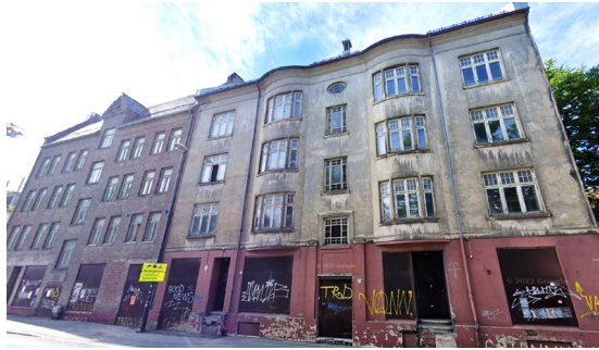
Figure 5-3: Photo of Elgeseter Street 4 and 6. (Google Street View, 2022)
