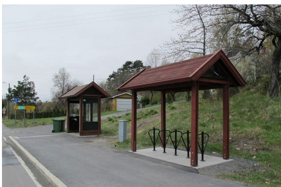
Figure 5-13: Photo of sheltered bus station and bicycle parking. (Statens Vegvesen, u.d.)
