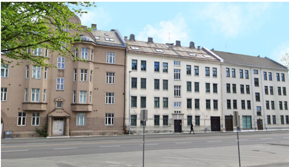
Figure 8: Photo of Elgeseter Gate 35, 37, and 39 today.
