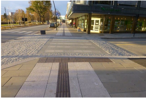
Figure 5-9: First photo of street in Hamar showing markings on sidewalks for the visually impaired. (Statens Vegvesen, u.d.)
