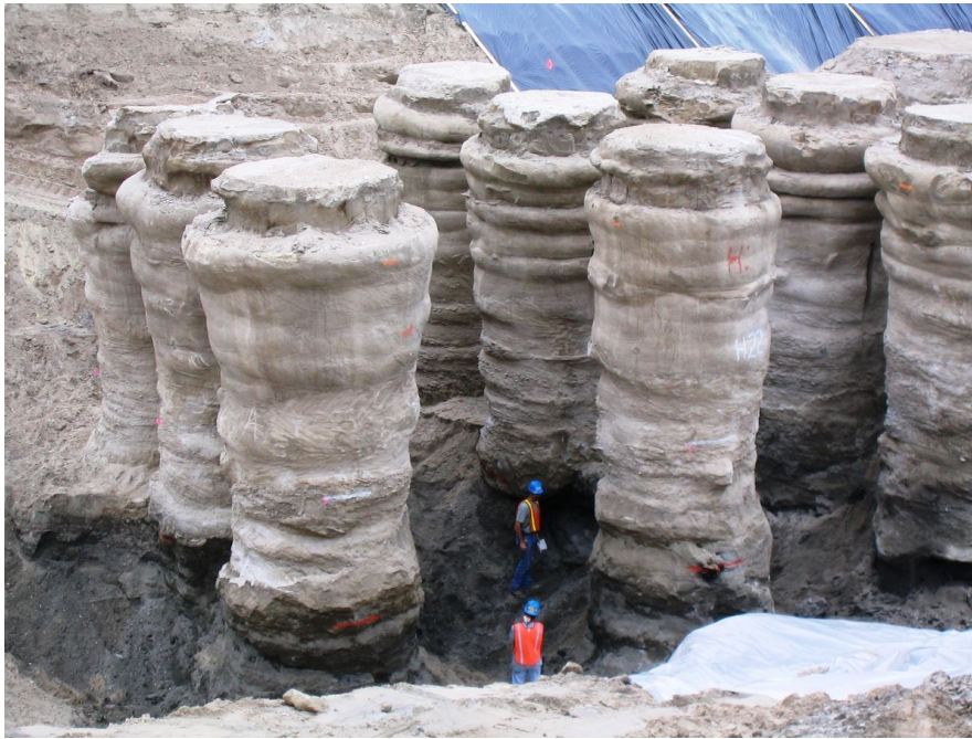
Figure 1.2: Picture of jet grouted columns [11].
