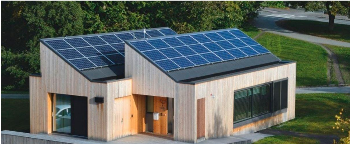
Figure 3.1: ZEB Living Lab at NTNU in Trondheim. Image source: Sintef, "ZEB Living Lab". Accessed via: https://www.sintef.no/laboratorier/living-lab/
