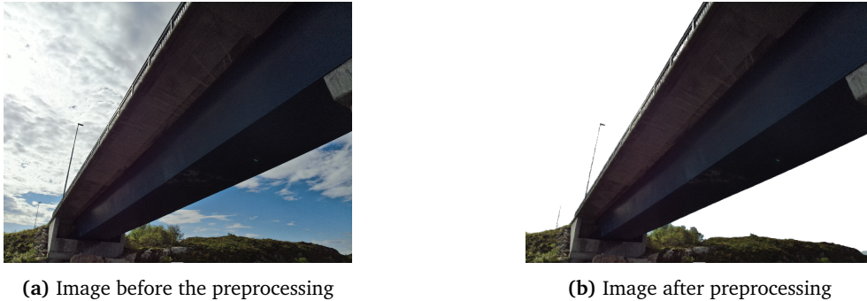
Figure 1.4: The goal of a sky network would be to remove unimportant pixels from images to have less disturbances for the Mask R-CNN.
