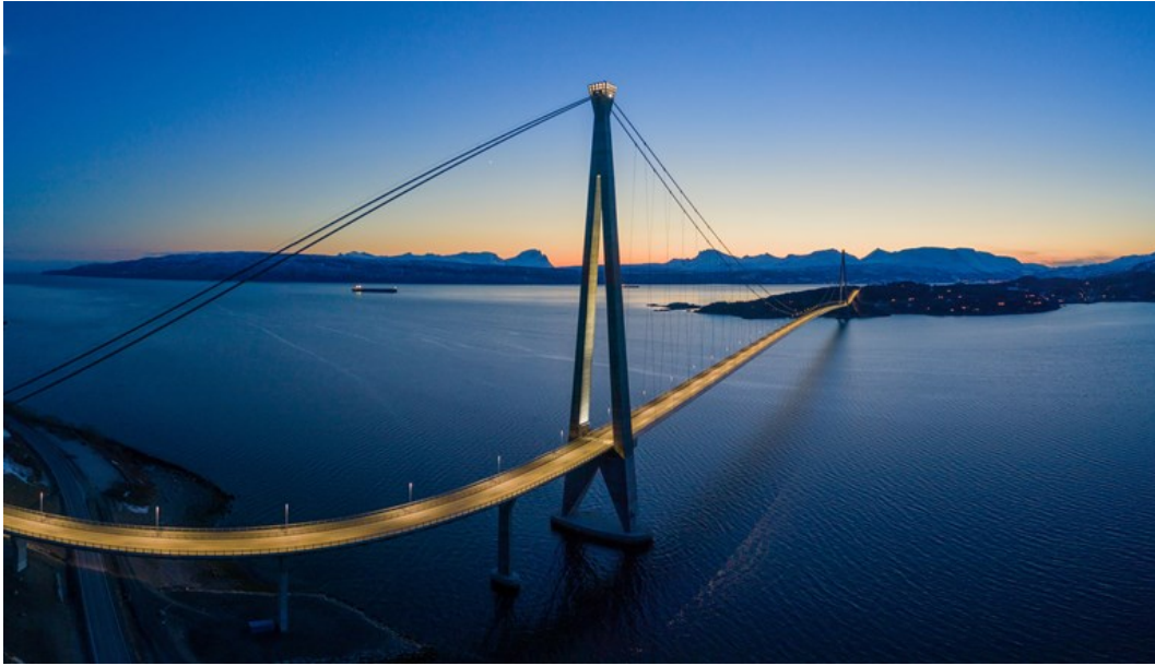
Figure 5: The Hålogaland Bridge viewed from the South-East, photo from Statens Vegvesen [50].
